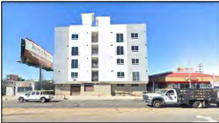
Photo 3: View of the eastern portion of the project site along Van Nuys Boulevard.
