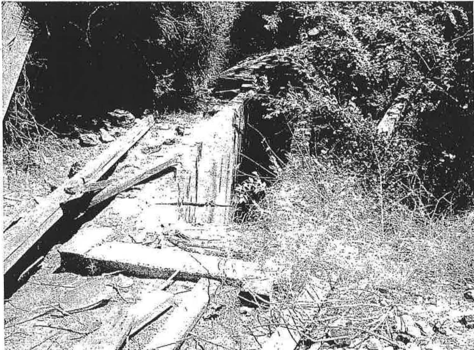
Photo 6: View east, entrance to subterranean well pump house.
