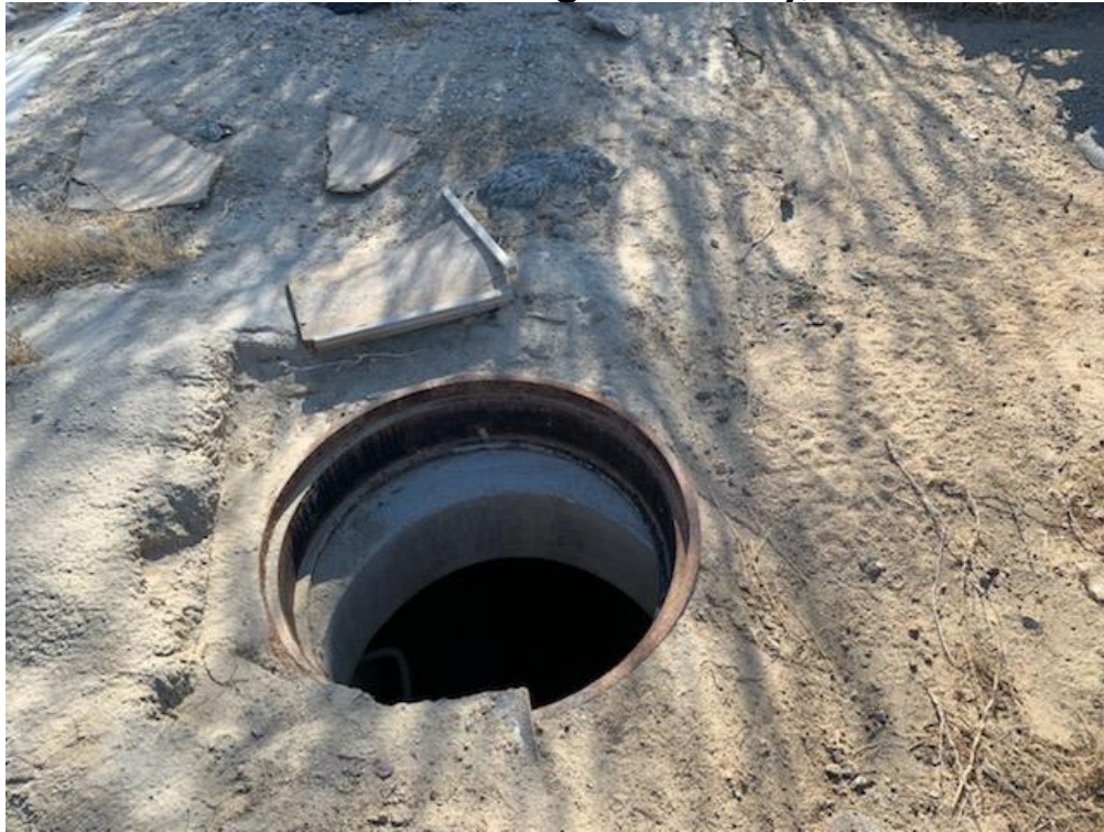
25. View open utility manhole on northeast portion of property.
