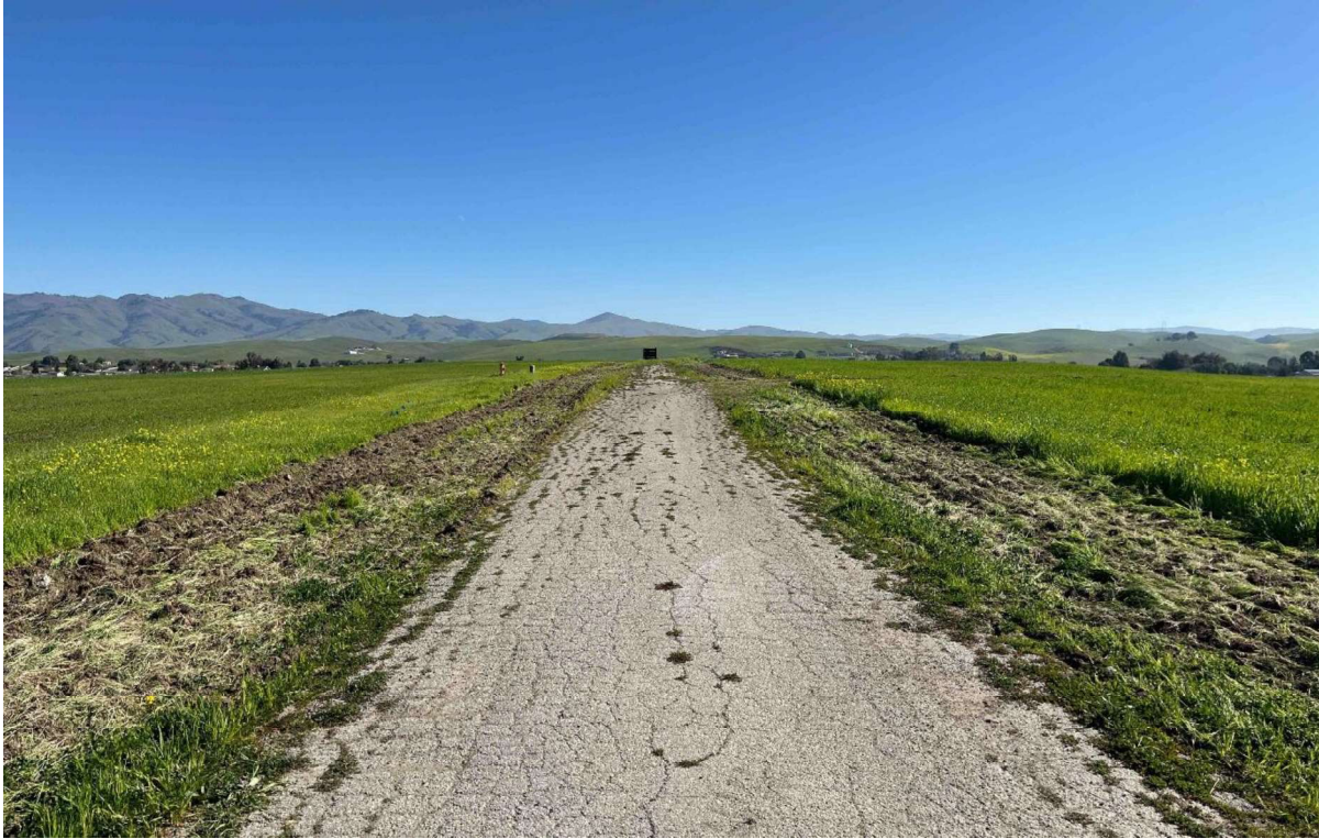
Photograph 3 Cement Road to Transformer Box, Facing East
