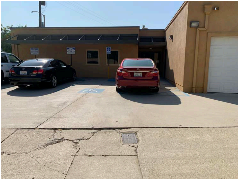
Photo 6 – Southerly view of the northern entrance to the building.
