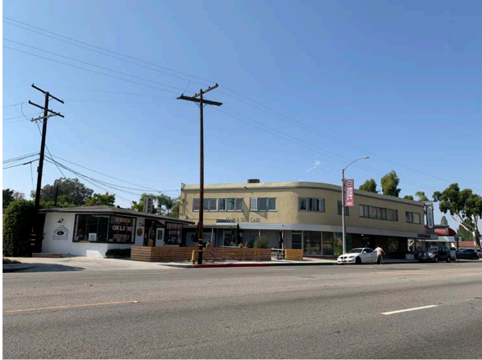
Photo 15 – Adjacent site to the north (4121-4129 Long Beach Boulevard) across the alleyway.
