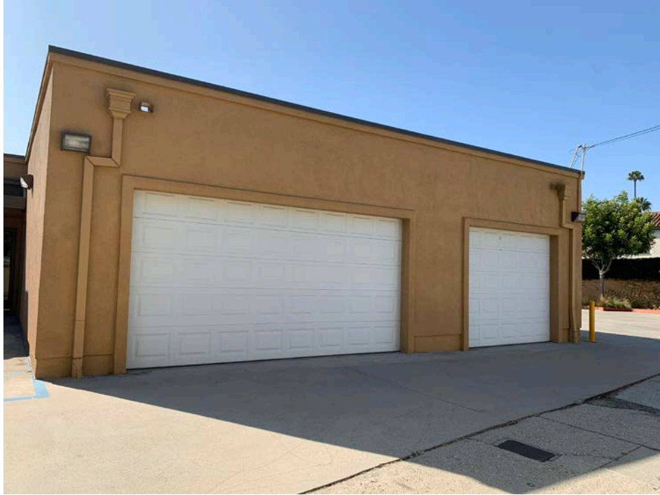
Photo 5 – Three-car garage attached to the northwestern corner of the building.
