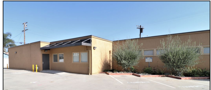
West elevation, view northeast (11/5/21). Note metal shade structure.
