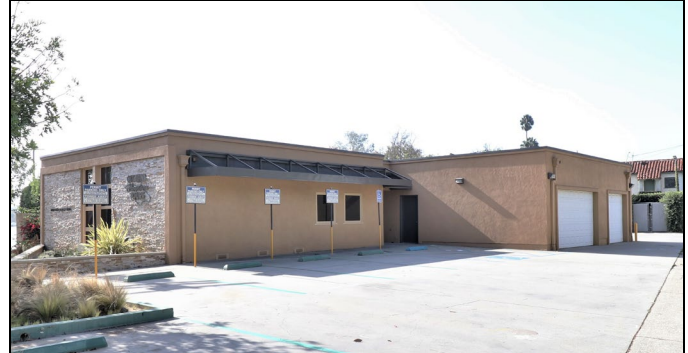
East and north elevations, view southwest (11/5/21). Note metal shade structure.
