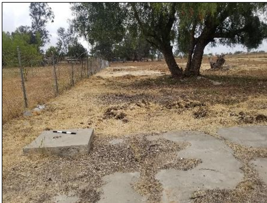
Figure 13. Overview of Frontage-Site-001, Feature 2
