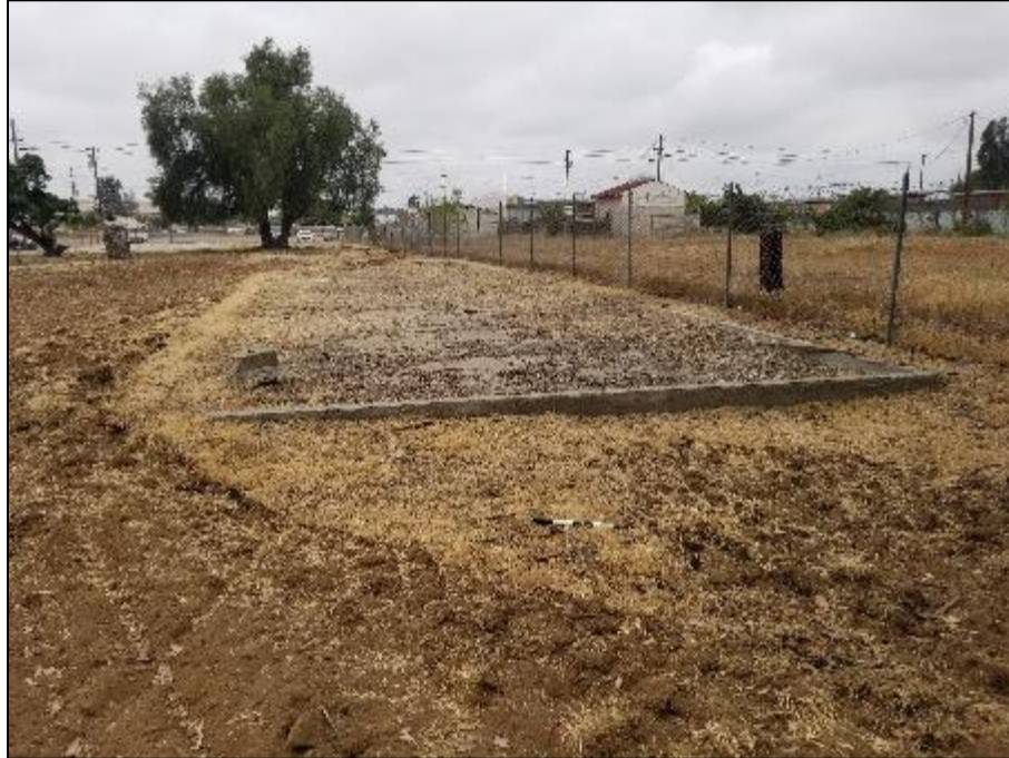
Figure 14. Overview of Frontage-Site-001, Feature 4
