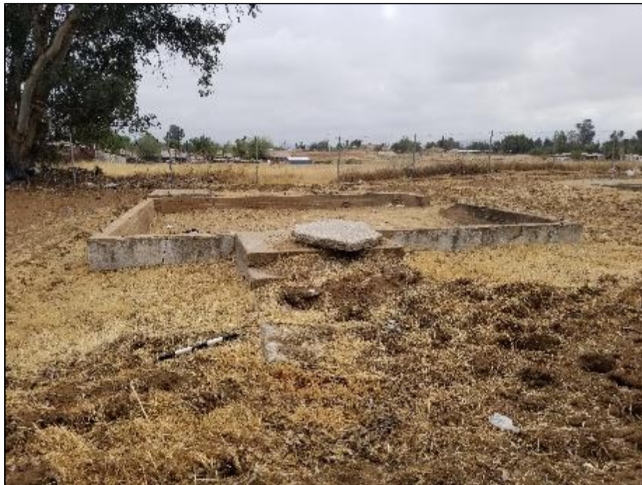
Figure 15. Overview of Frontage-Site-001, Feature 13
