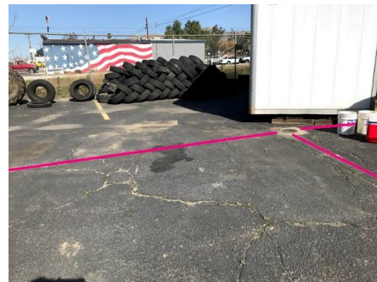
Photo showing where unknown piping was located either with an EM pipe locator or GPR.
