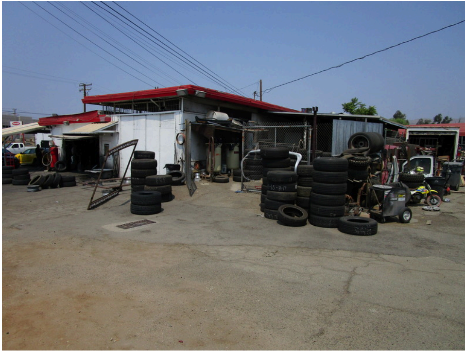
13. South side of P&B Tires building at subject property
