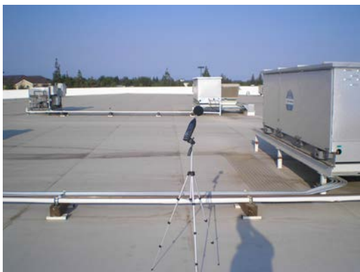
Rooftop Mechanical Equipment Noise Measurement
