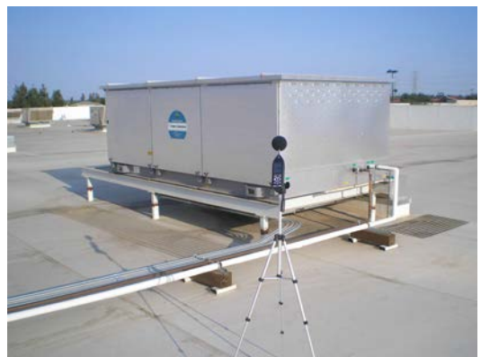
Rooftop Mechanical Equipment Noise Measurement
