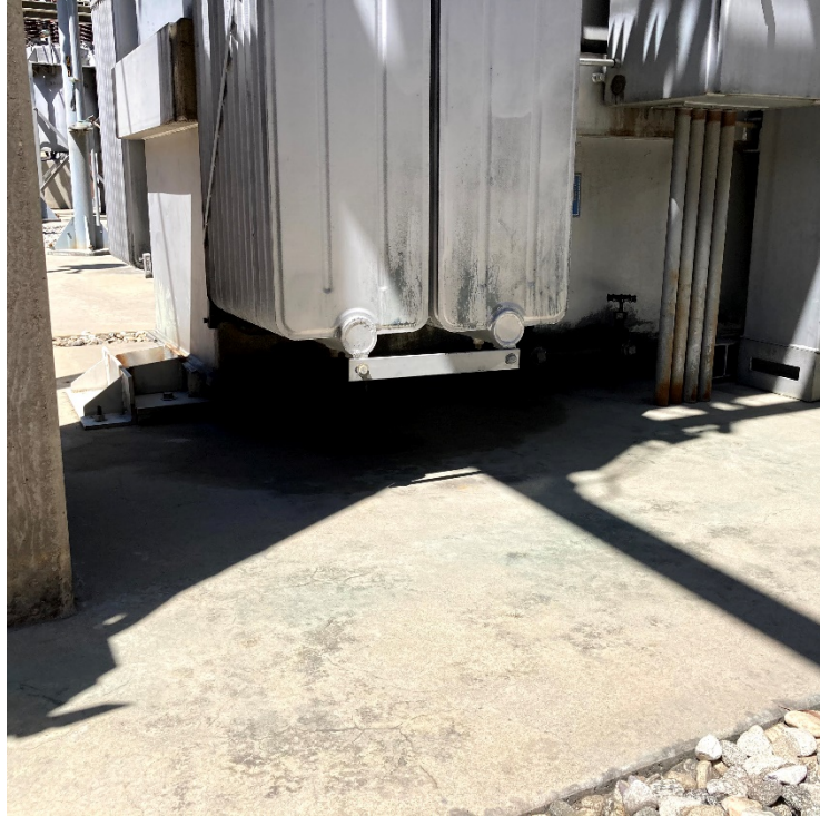
Photo 11: Concrete Wipe Sample Location C
