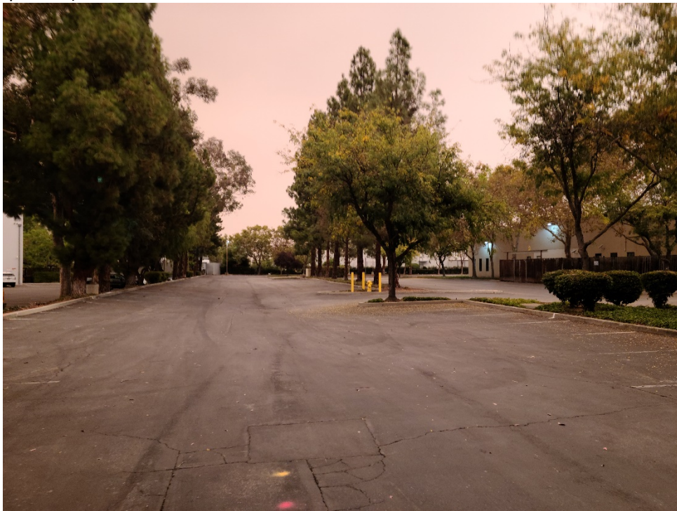
Photo 6: Looking northeast along northern border of Study Area (northern portion).
