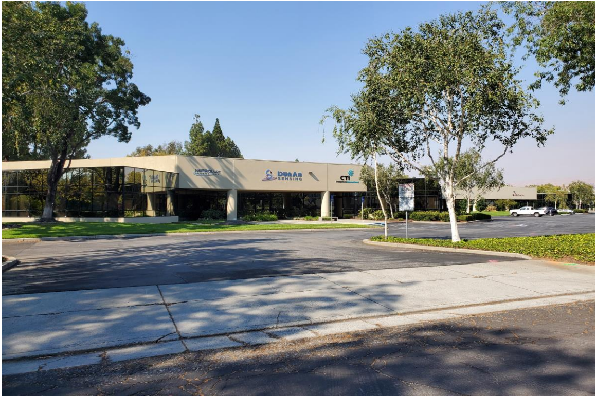
Photograph No. 1: View of site building from Concourse Drive, looking north
