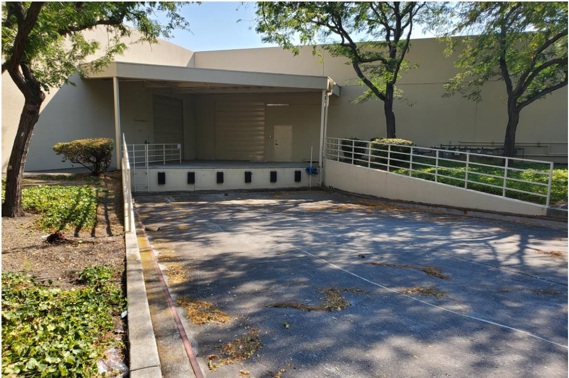
Photograph No. 16: Loading dock shared by 1959 and 1961 Concourse Drive.
