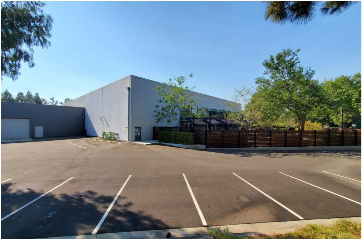
Photograph No. 18: Western adjacent facility (Blach Construction) viewed from site boundary, looking west.
