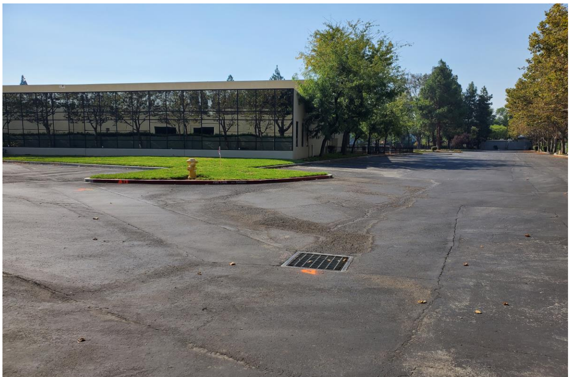
Photograph No. 14: Northeastern site parking area and typical stormdrain, looking northwest.
