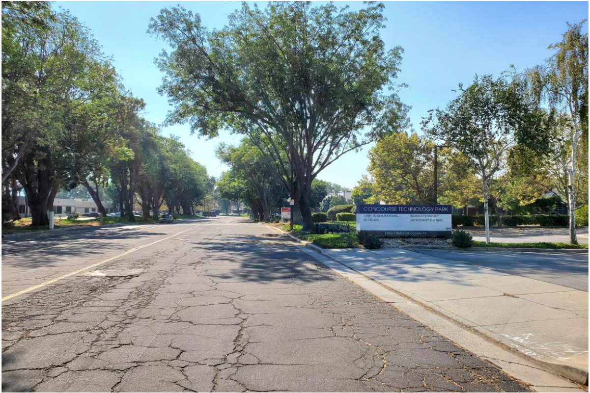
Photograph No. 21: Concourse Drive, looking west.
