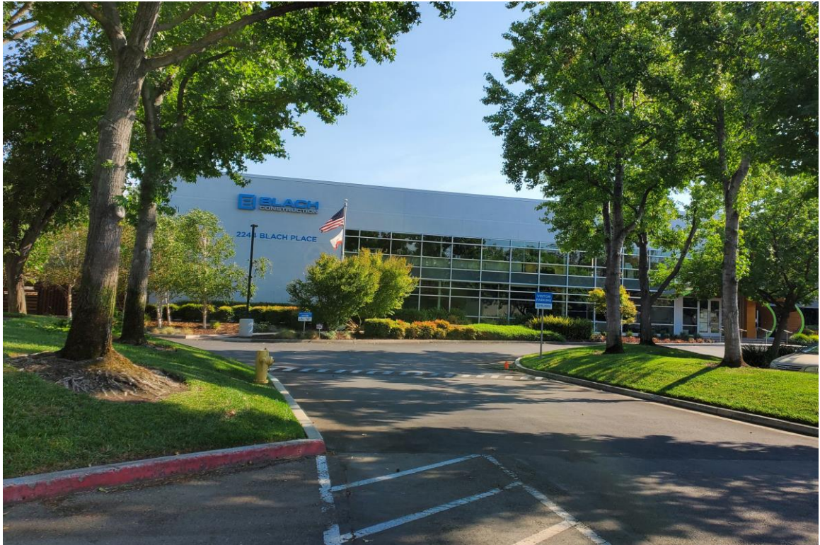
Photograph No. 19: Blach Construction main entrance.
