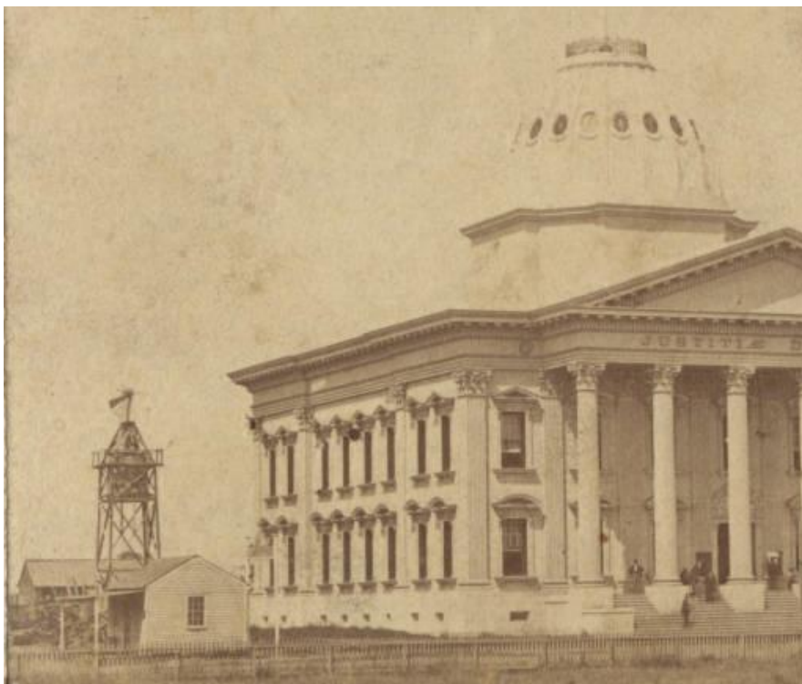
Figure 4. 1869 photograph of the first Santa Clara County Courthouse (courtesy of the Martin Luther King Jr. Library, California Room).
