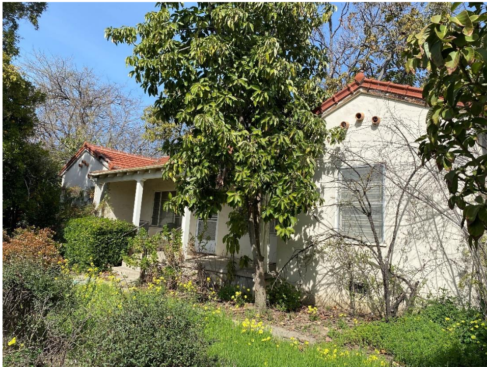
Figure 42. West elevation, facing northeast.
