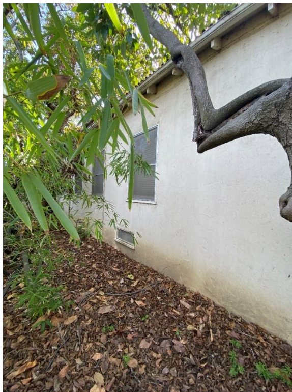
Figure 46. East elevation of the ca. 1920 house, facing south.
