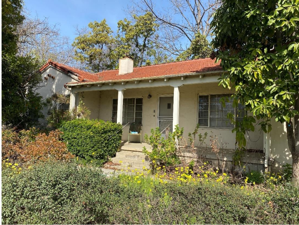
Figure 43. West elevation, facing northeast.
