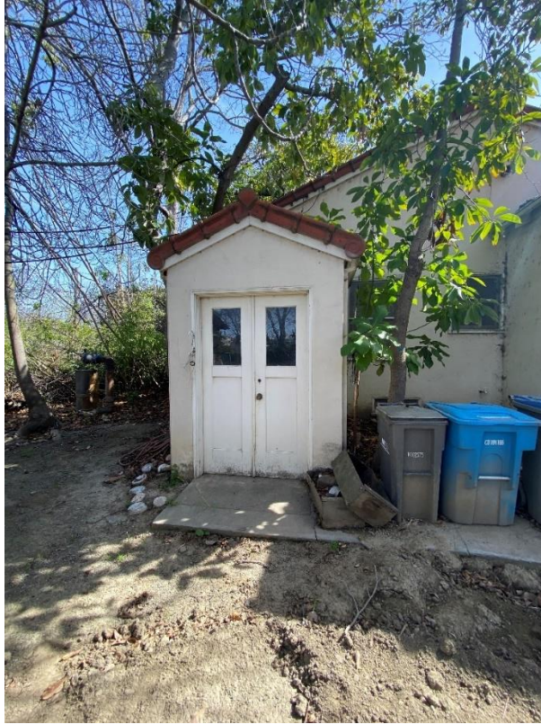
Figure 45. Photograph showing the projecting gable entry into the basement where the Sakauye family, as well as other Japanese Americans, stored their belongings during their internment from 1942 to 1945.
