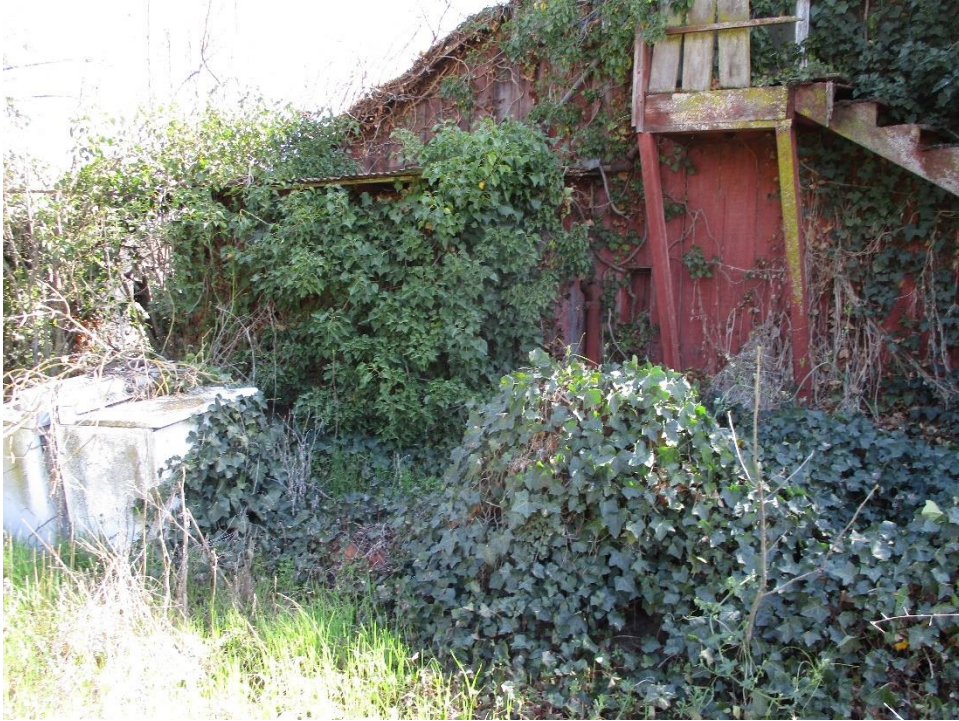
Figure 39. Photograph showing the north elevation, facing south.
