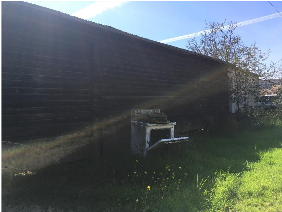
Figure 60. Photograph showing the north elevation of the ca. 1975 barn, facing west.
