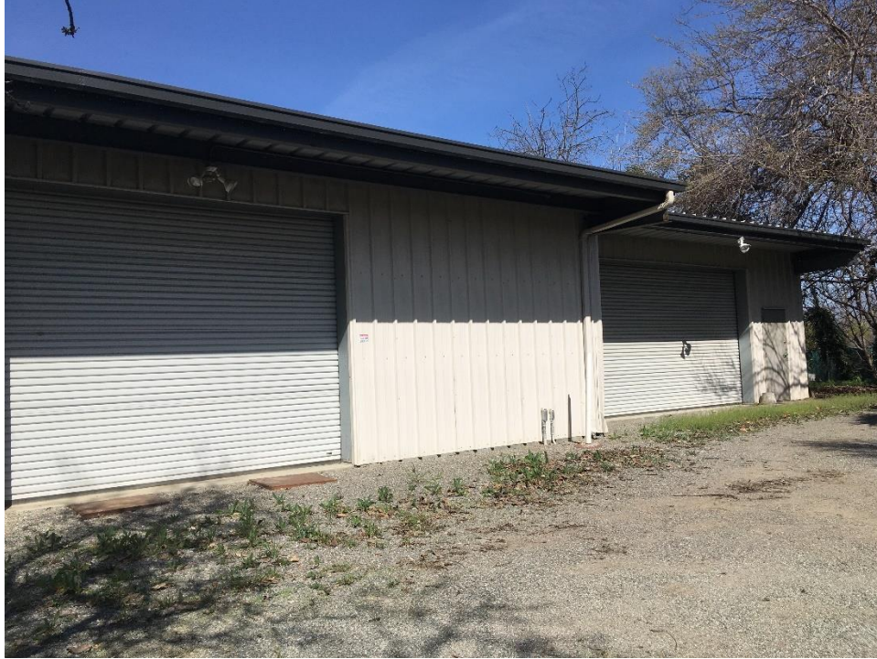
Figure 52. Photograph showing the south elevation of the 2004 storage building, facing east.
