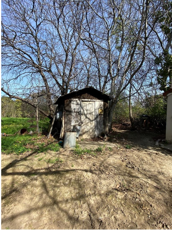
Figure 53. Photograph showing west elevation of the ca. 1930 shed.
