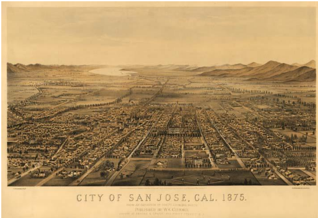
Figure 5: 1875 Bird's eye view of San Jose, facing north.
