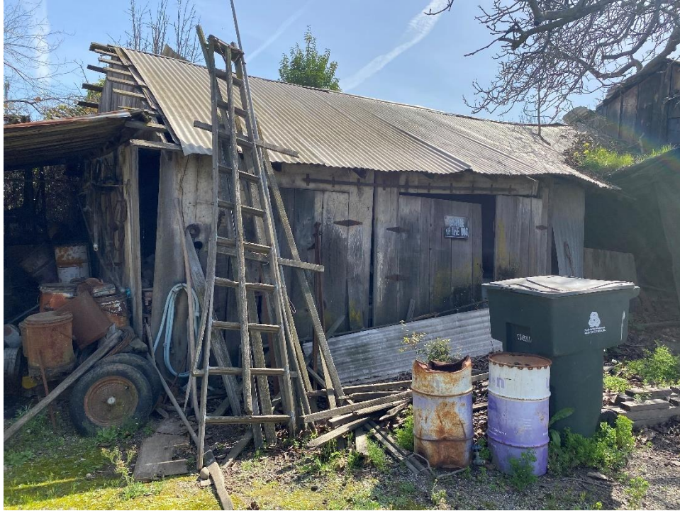
Figure 50. Photograph showing the north elevation of the linear form, facing south.
