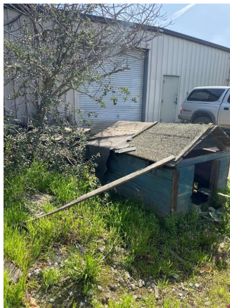
Figure 62. Photograph showing the ca. 1995 doghouse, facing southwest.
