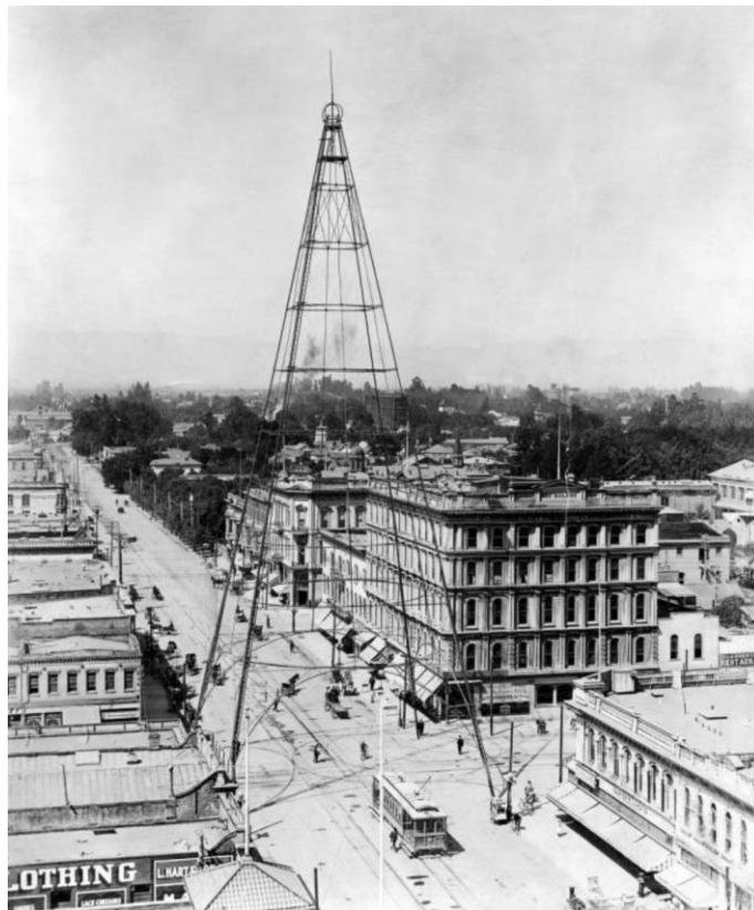
Figure 8. 1910 photograph of the San Jose Electric Light Tower (courtesy of the Martin Luther King Jr. Library, California Room).
