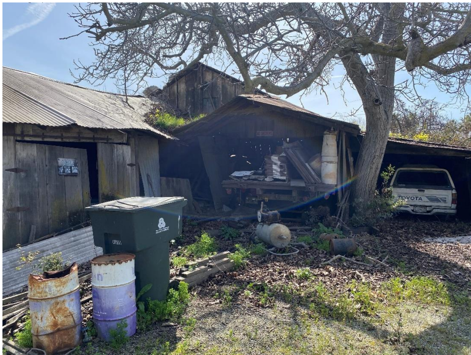
Figure 51. ca. 1910 barn, facing west.
