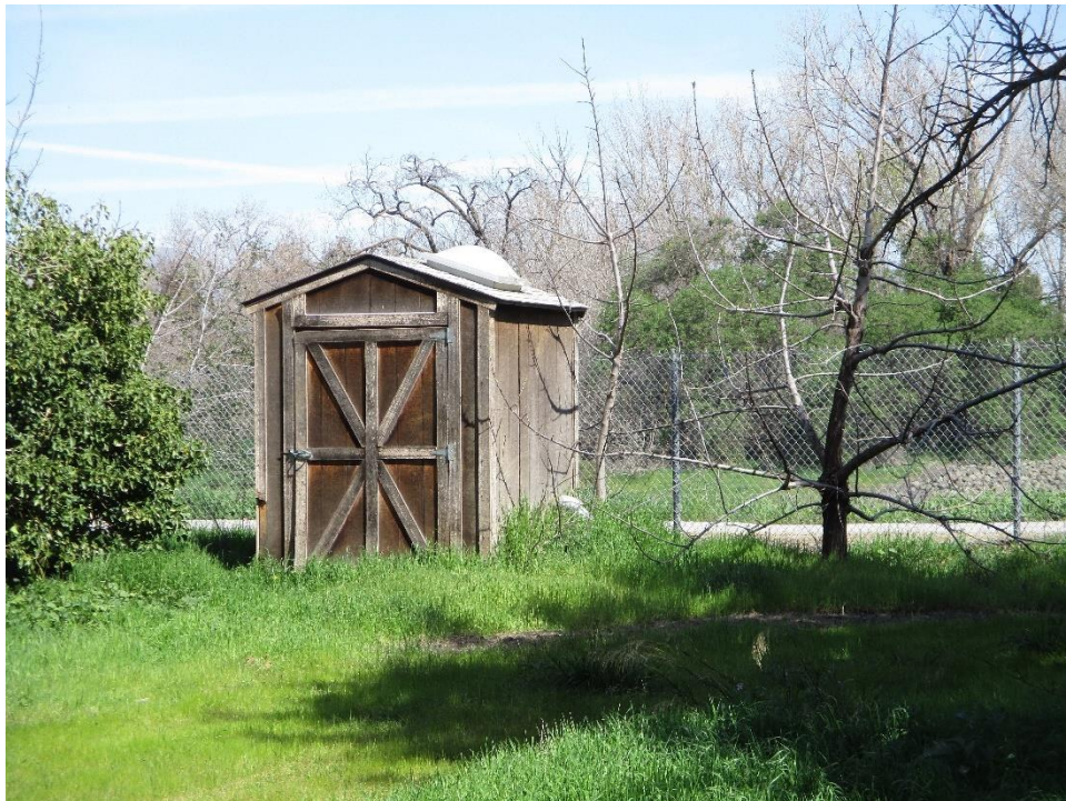
Figure 40. West elevation, facing east.
