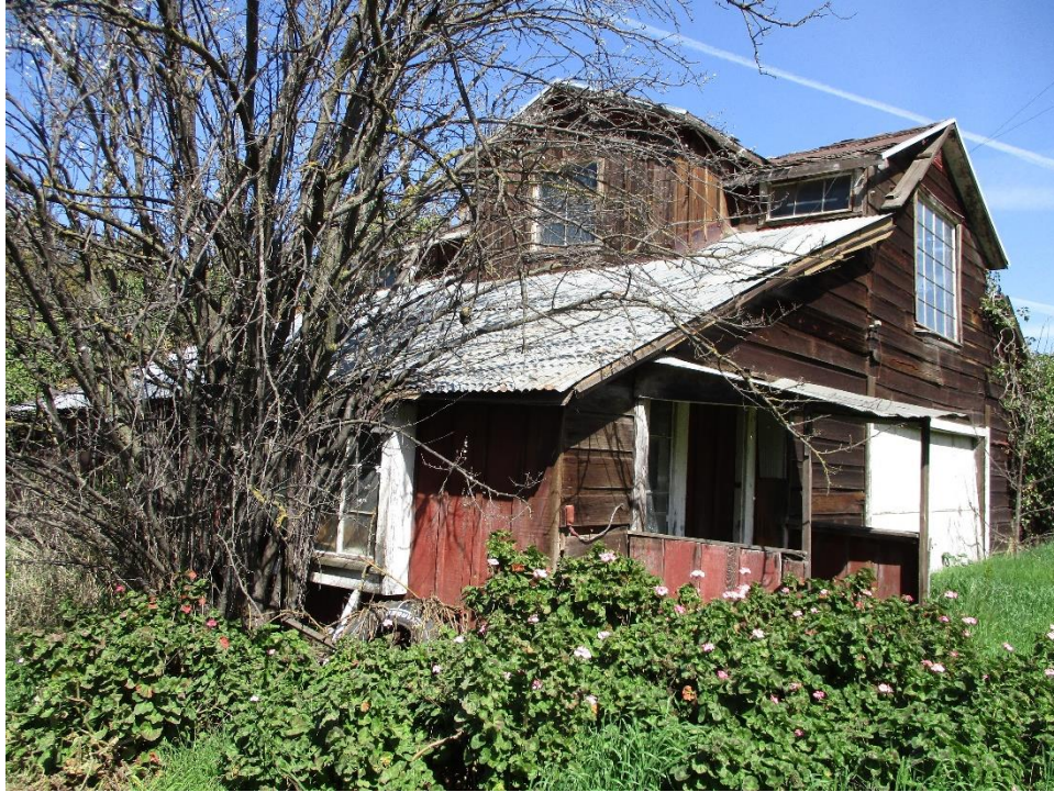
Figure 37. ca. 1890 barn showing west and south elevations, facing east.
