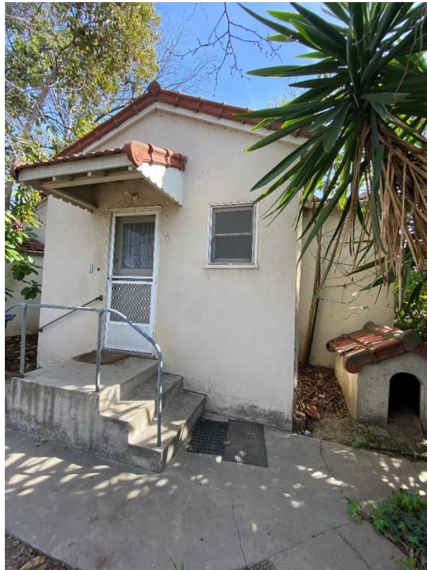
Figure 44. North elevation, showing the side entrance to the house.
