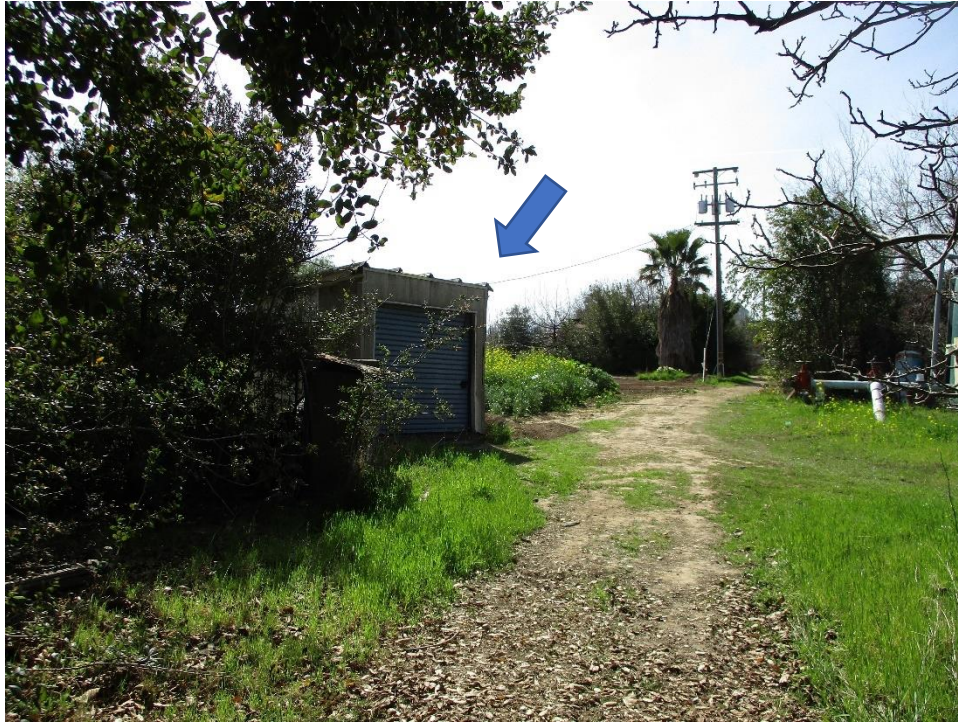
Figure 41. Photograph showing the 2005 container shed (see blue arrow), facing west.
