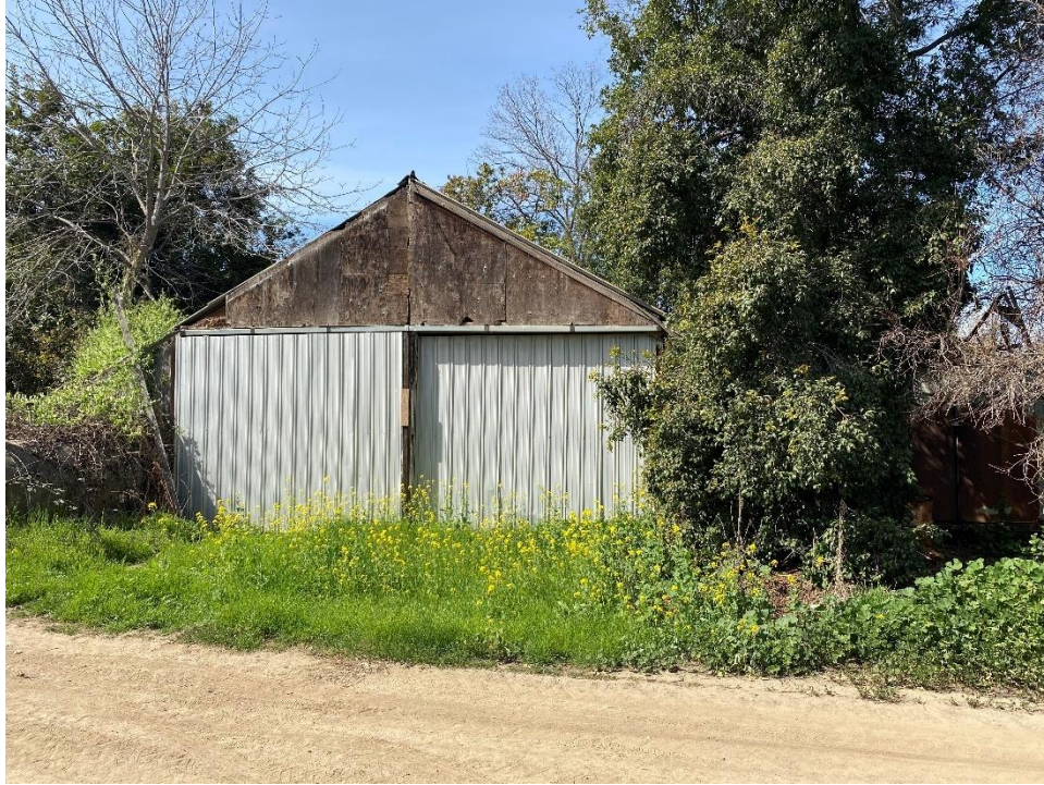
Figure 56. Photograph showing the south elevation of the ca. 1955 barn, facing north.
