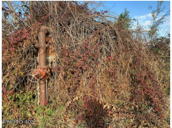
PHOTO 10 FORMER WELL SHED AND PUMP
