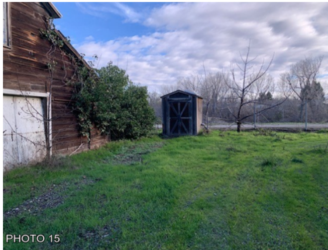
FORMER PUMP SHED
