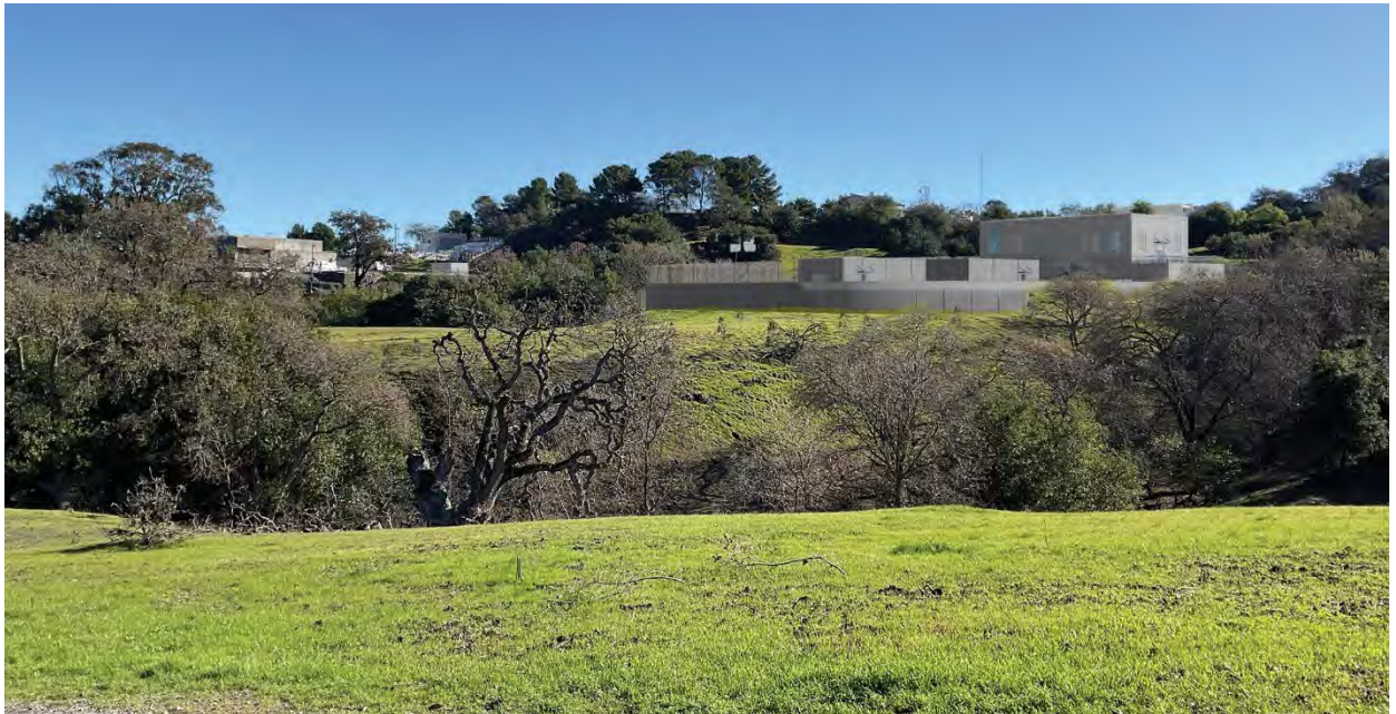
After Construction - gravity thickeners, thickened solids pumping plant, and solids dewatering building partially visible
