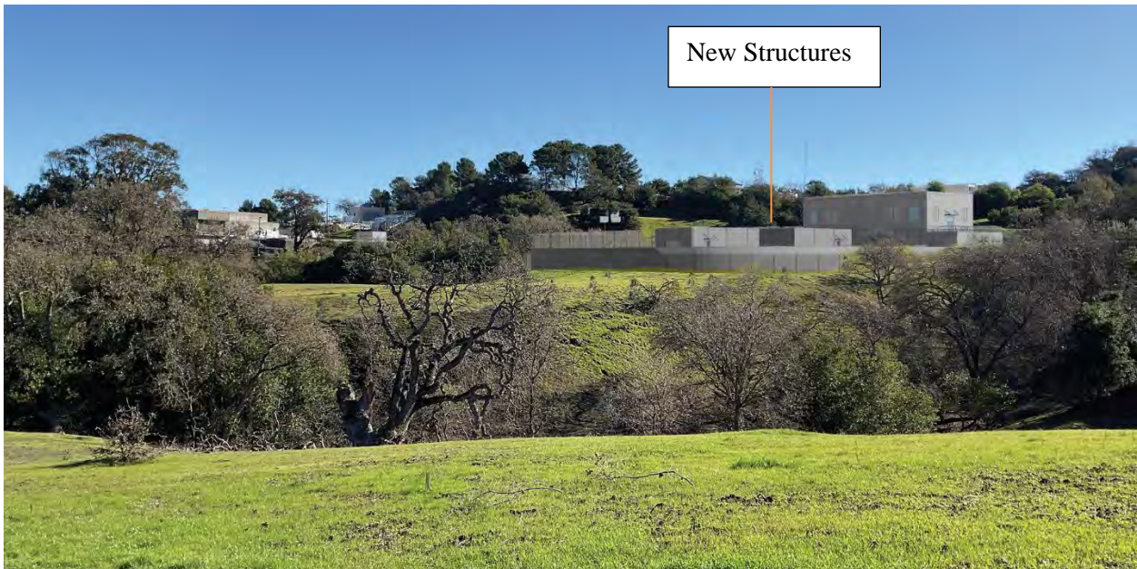
After Construction - Gravity thickeners, thickened solids pumping plant, and solids dewatering building partially visible
