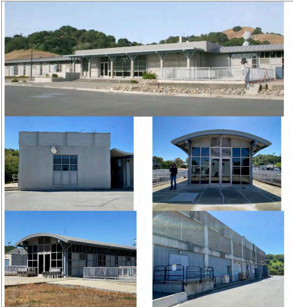
Figure 2-9: Existing Buildings at the Walnut Creek WTP
