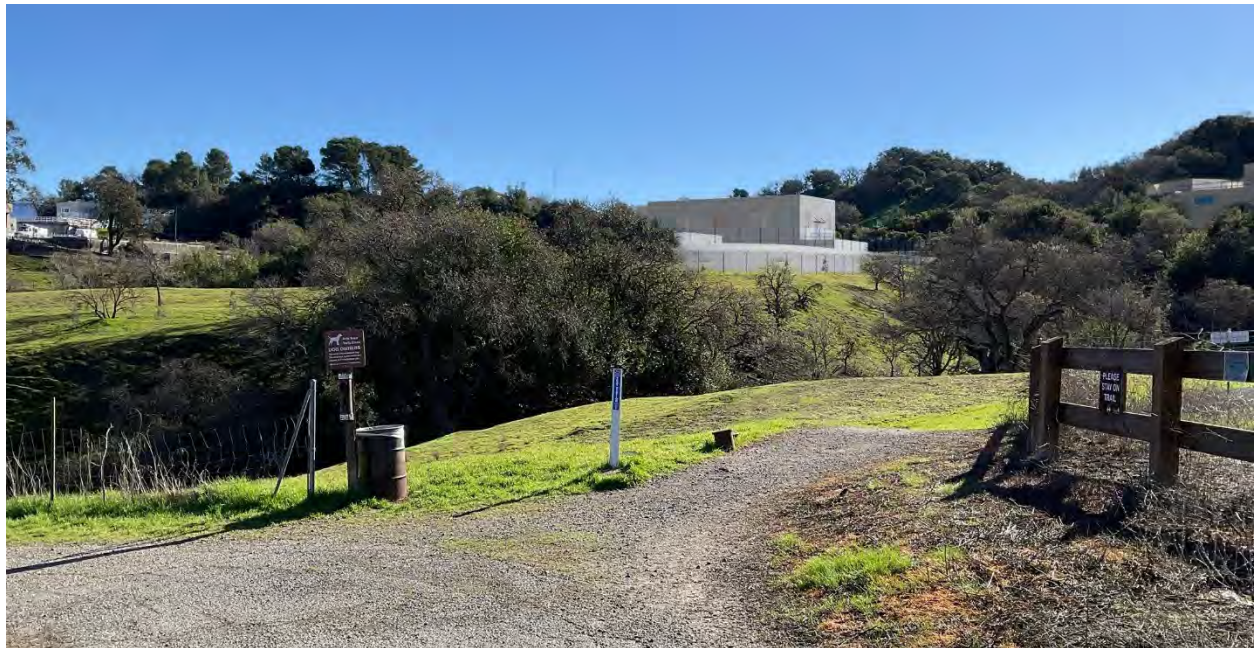
After Construction - Gravity thickeners, thickened solids pumping plant, solids dewatering building, liquid oxygen storage area and electrical building
