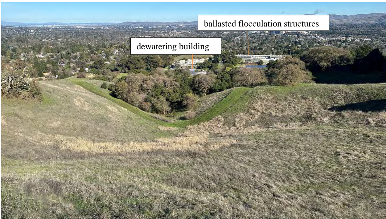
After Construction – Ballasted flocculation structures and dewatering building partially visible
