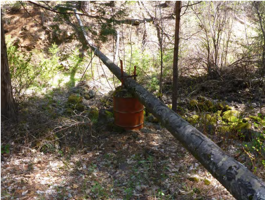
Existing pipeline crossing at Paynes Creek. April 29, 2021.
