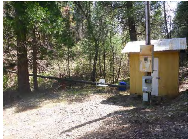
Photo 1. Transmission Main Connection to Existing Well
