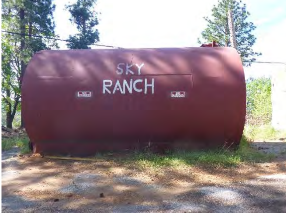
Photo 4.1-1. Existing 18,000-gallon tank to be demolished
