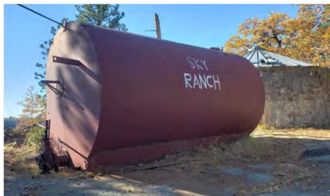
Photo 4. 18,000-Gallon Water Tank; Stone Tank in the Background.
