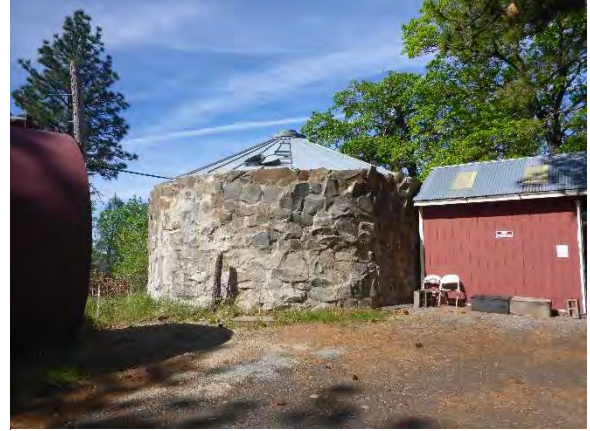
Photo 4.1-2. Abandoned 50,000-gallon stone tank and booster pump station to be demolished
