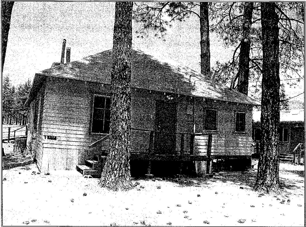
Figure 13: Views of the Administration (Office) Building.
