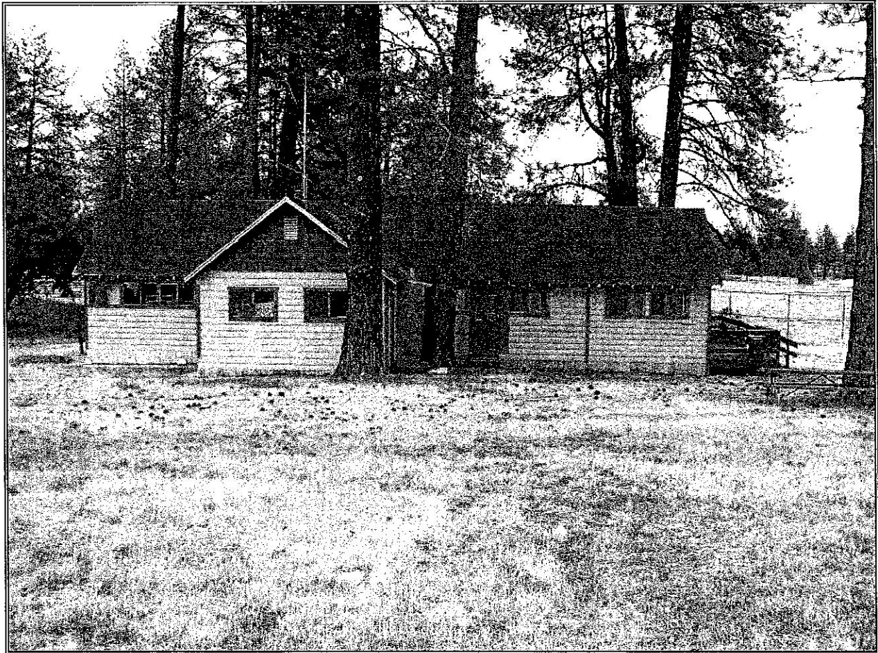
Figure 26: West side view of Cabin 18 showing room addition.
