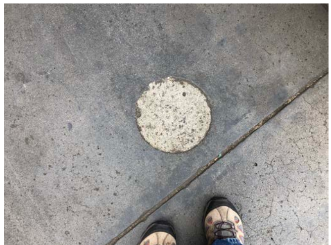
24. Capped subsurface boring near clarifier
