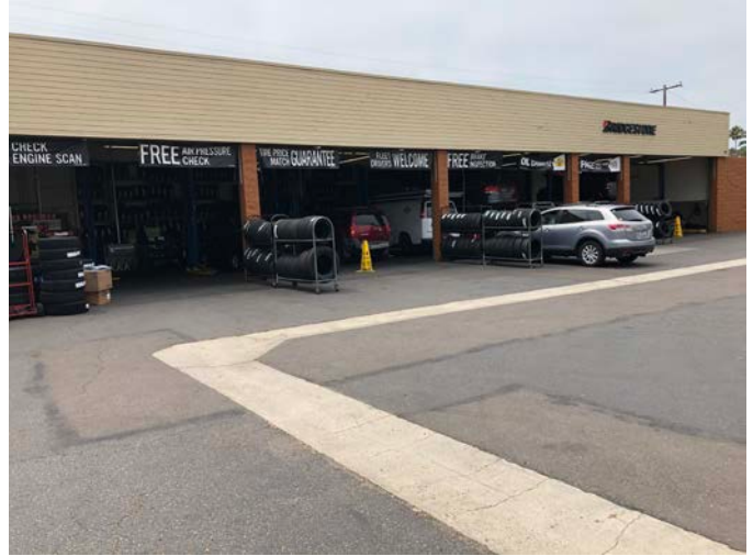
2. Front face of auto repair
