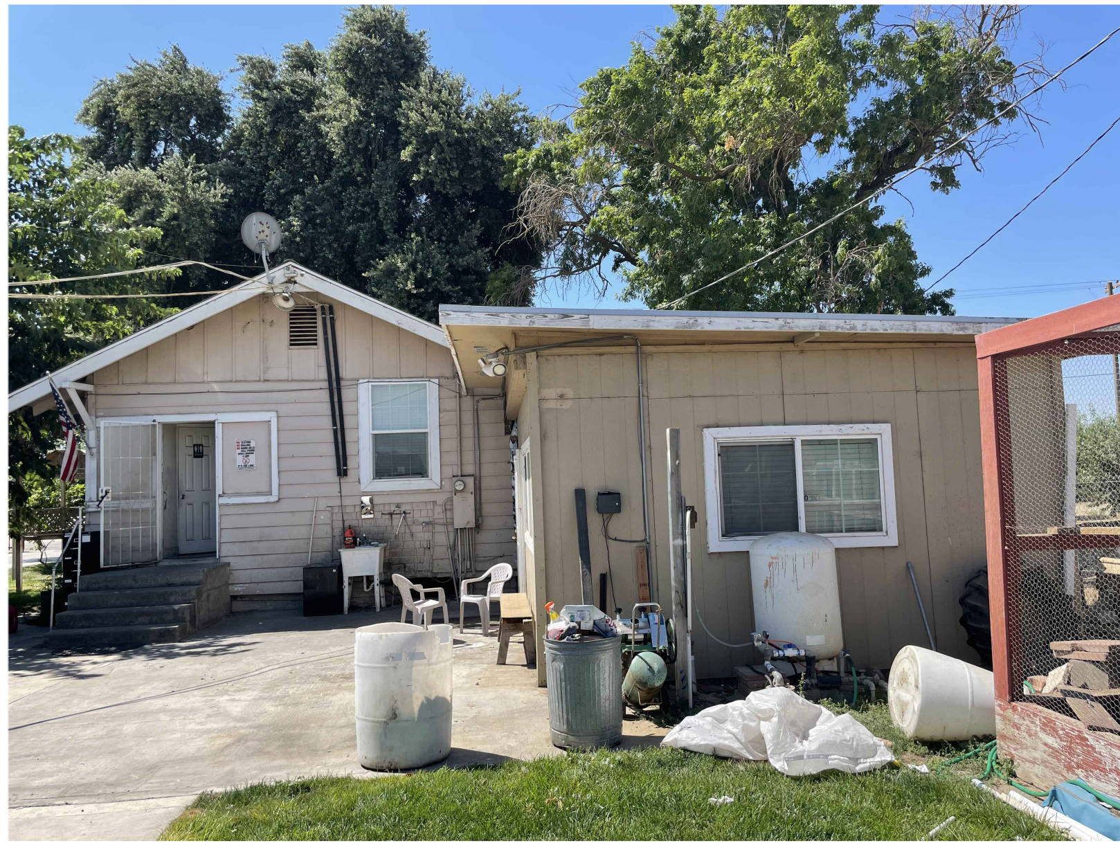
EXISTING OFFICE - NORTH
