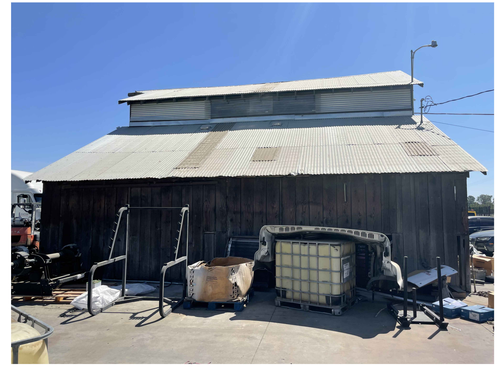
EXISTING SHOP - WEST
