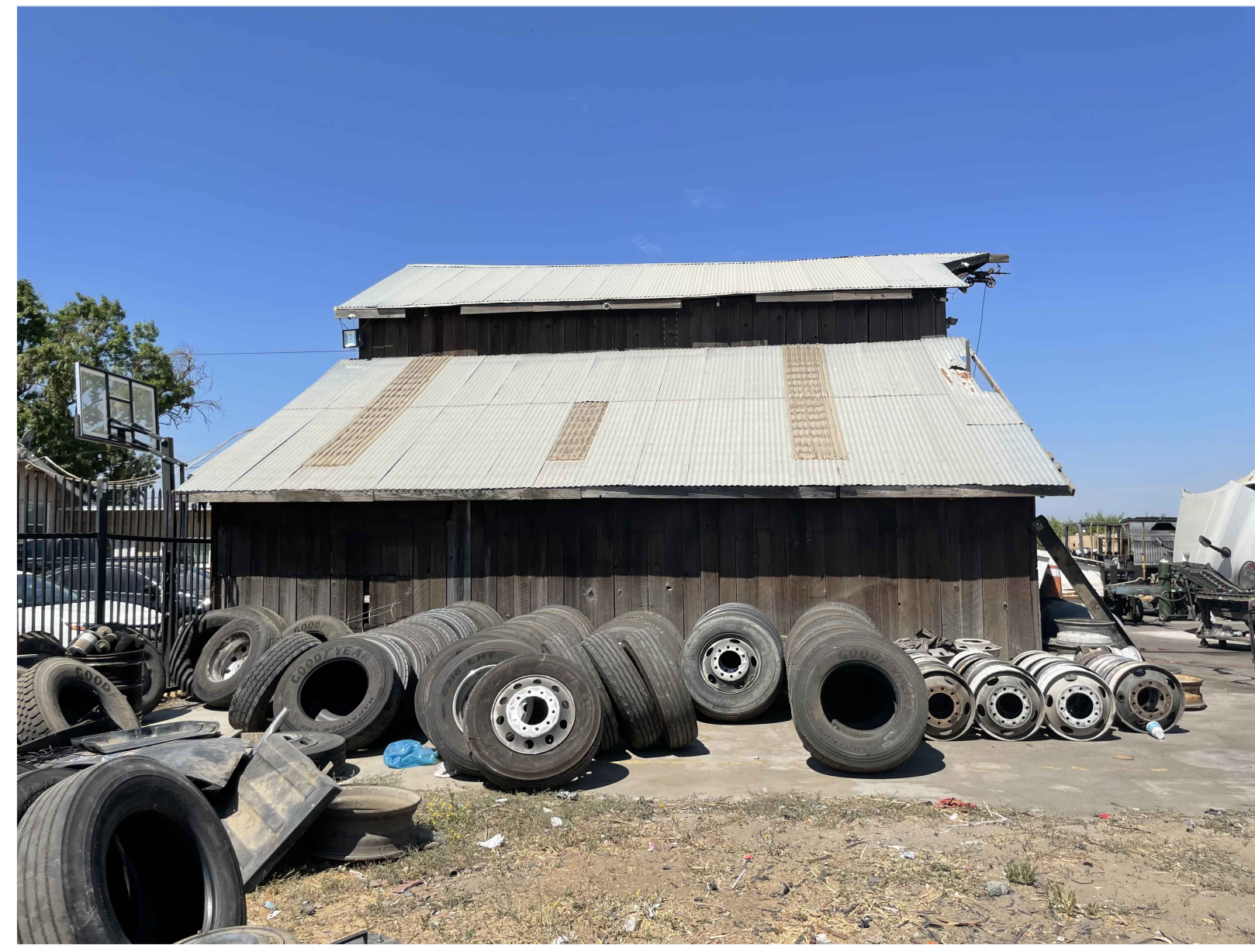
EXISTING SHOP - EAST
