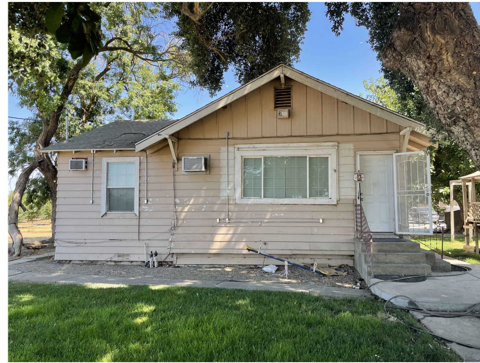
EXISTING OFFICE - SOUTH
