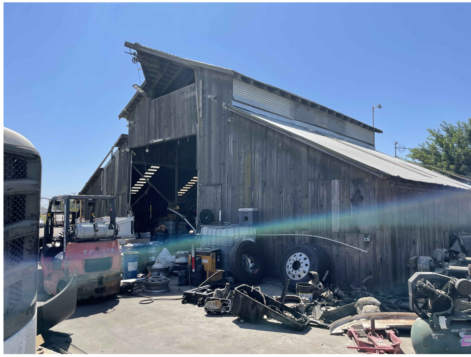
EXISTING SHOP - NORTH
