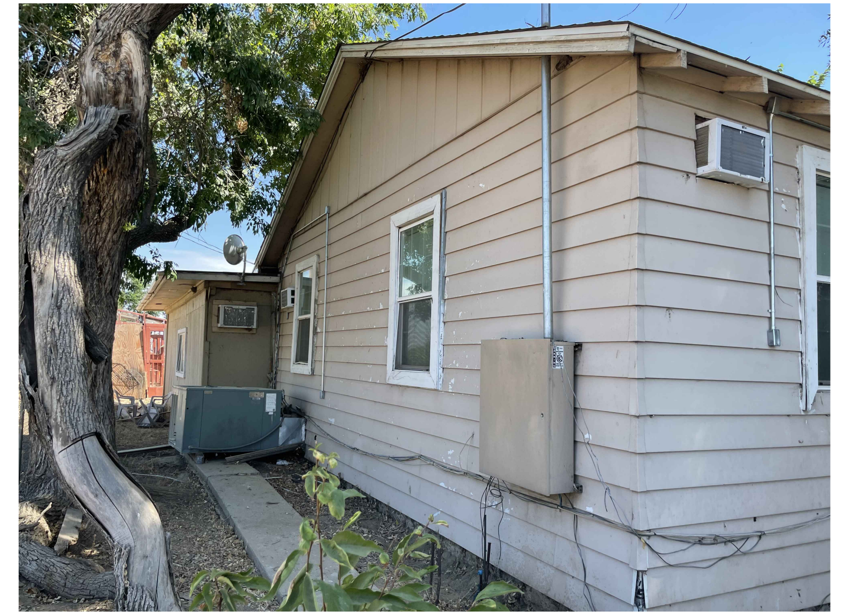
EXISTING OFFICE - WEST
