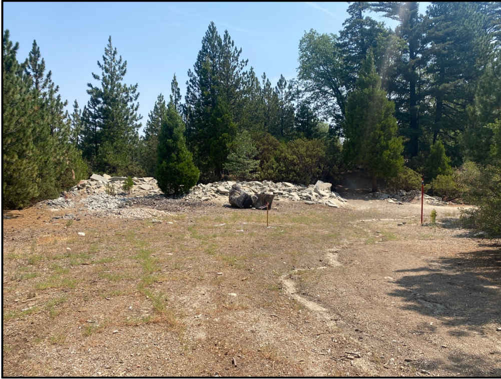
Plate 3.2–3: Overview of the piles of concrete rubble in the center of the project, facing north.
