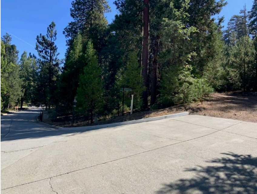
Photo 1. Paved road providing access to residential sites, the club house, and maintenance buildings.
