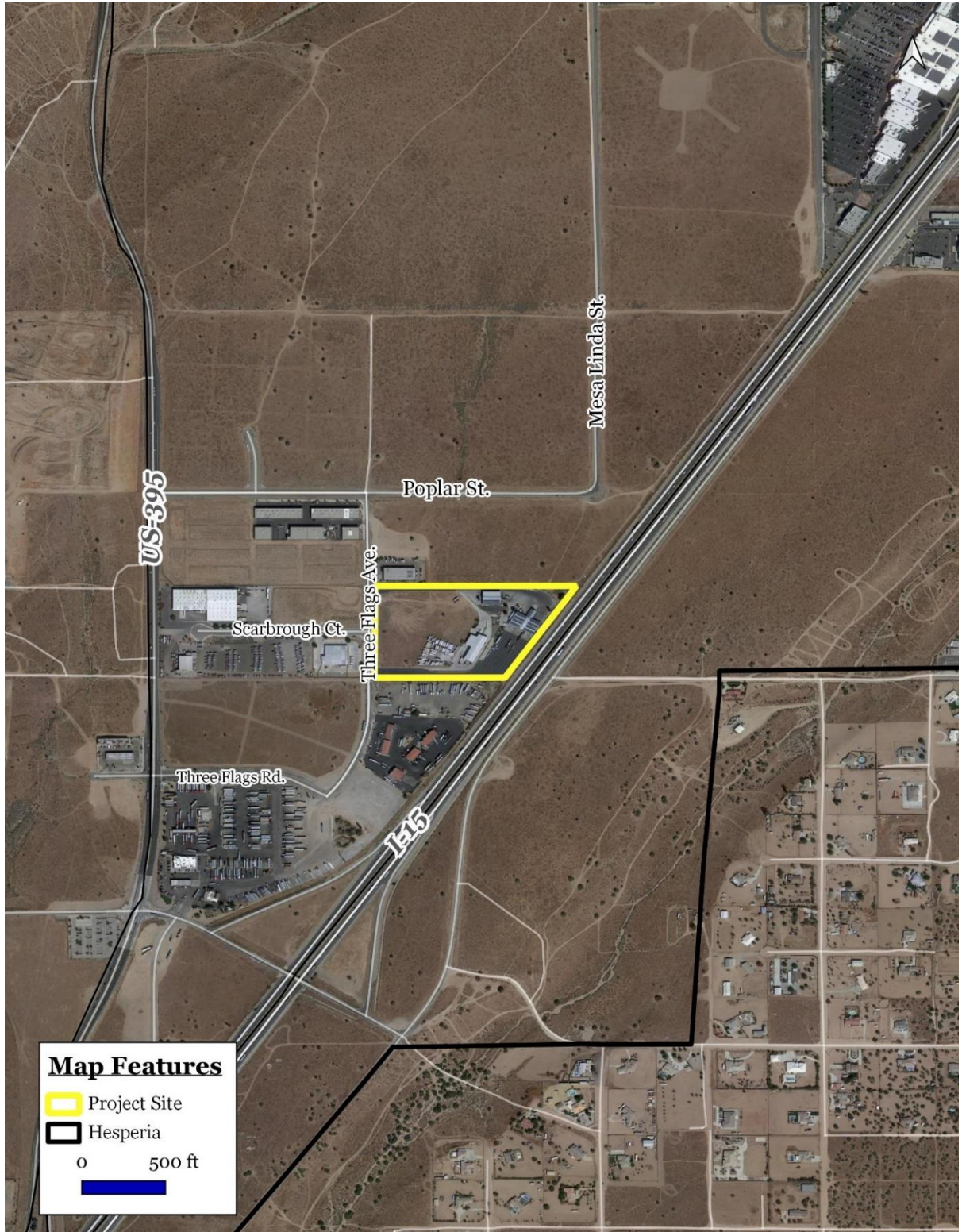
EXHIBIT 2-4 AERIAL IMAGE OF PROJECT SITE SOURCE: BLODGETT BAYLOSIS ENVIRONMENTAL PLANNING
