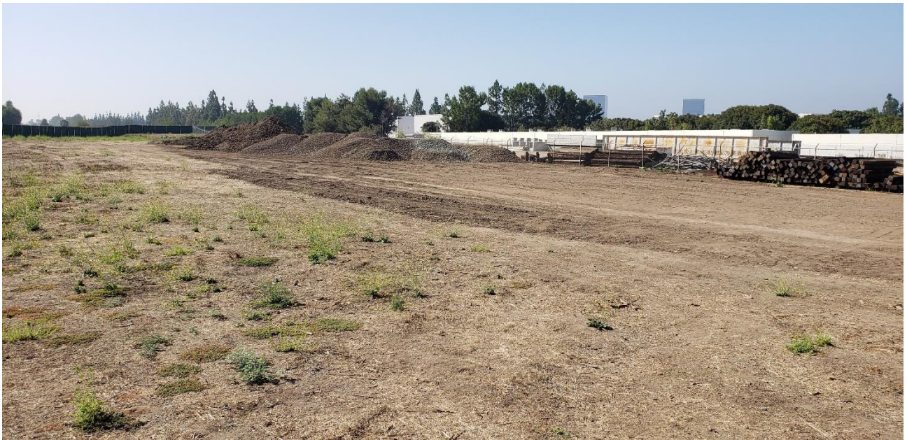
Photo 6. South-facing view of railroad equipment and materials stored onsite.
