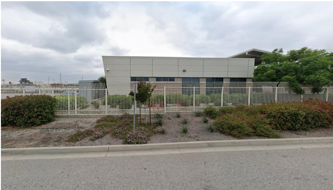
Figure 5.4-2 Existing Eastern Maintenance Facility, Exterior Building Materials
