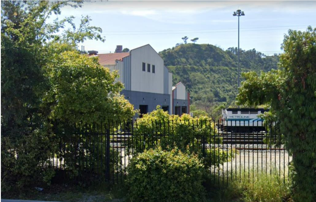
Figure 5.4-1 Existing Central Maintenance Facility, Exterior Building Materials
