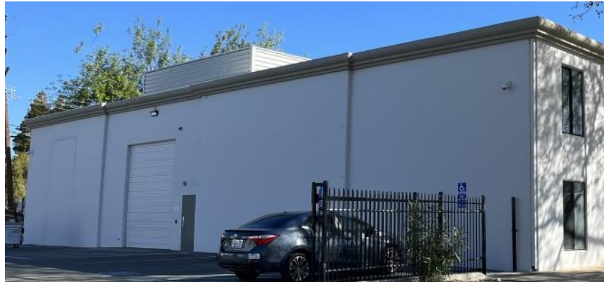
Figure 73. The east façade.
