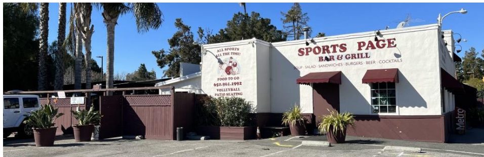
Figure 43. The east façade.
