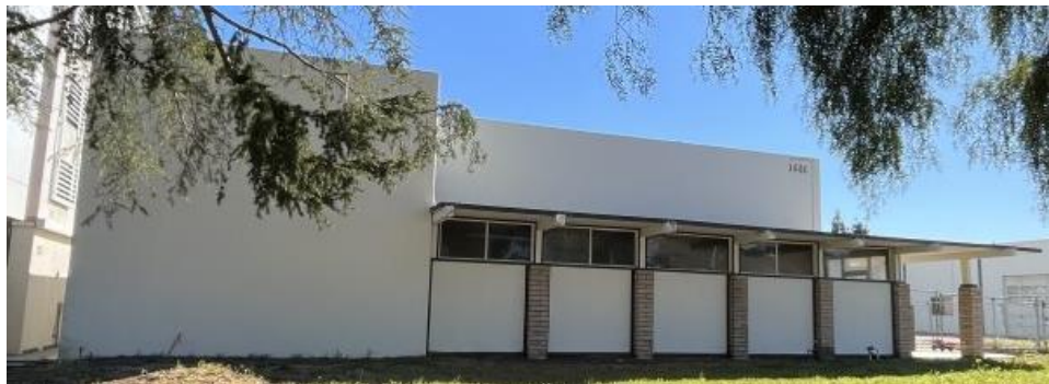
Figure 62. The west façade of 1601 N. Shoreline Boulevard.
