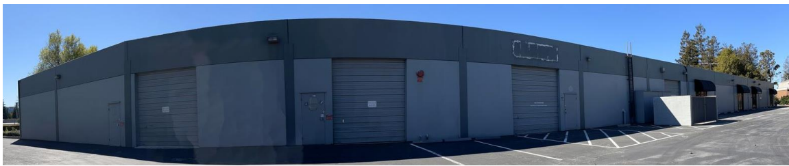
Figure 49. Building A, south façade.
