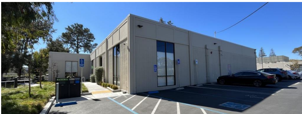
Figure 41. The north façade.
