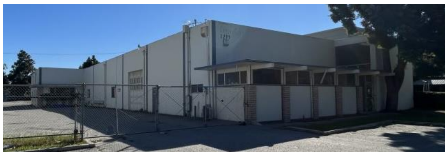
Figure 58. The north and west facades of 1599 N. Shoreline Boulevard.
