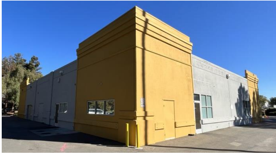
Figure 47. West and south facades.
