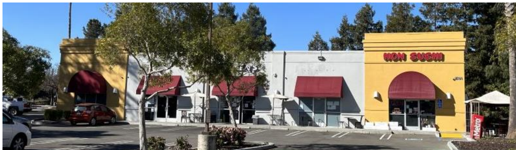
Figure 45. The east façade.
