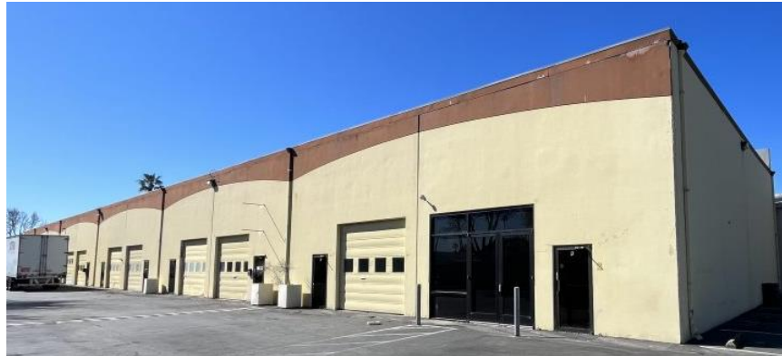
Figure 55. The east façade.
