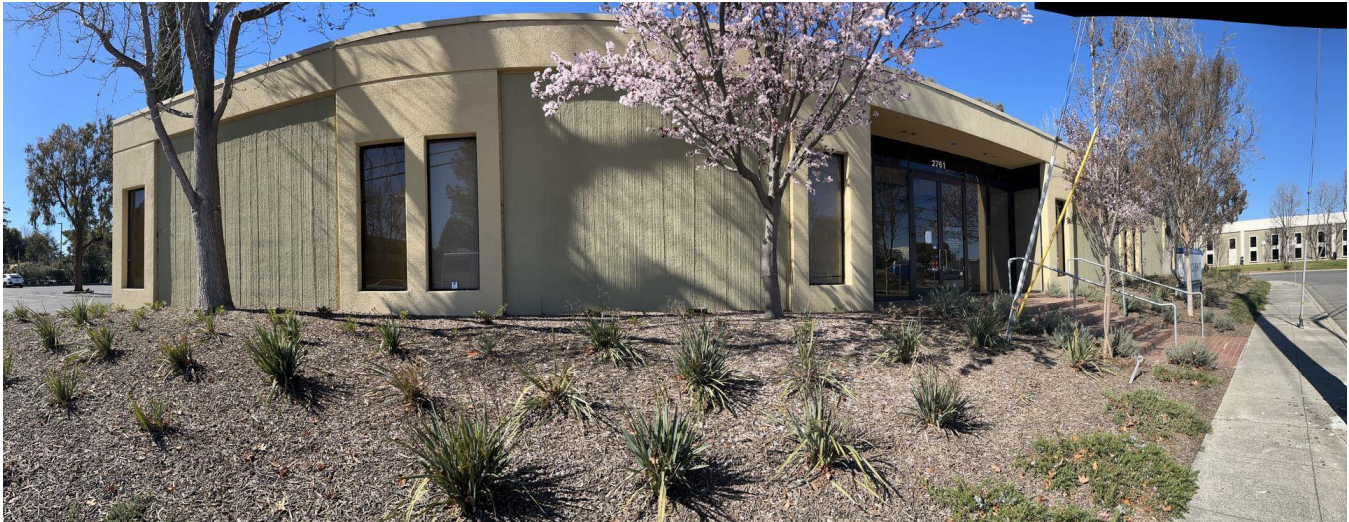
Figure 26. East façade of 2761 Marine Way.
