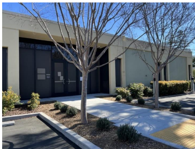
Figure 22. The west façade of 1161 San Antonio Road.
