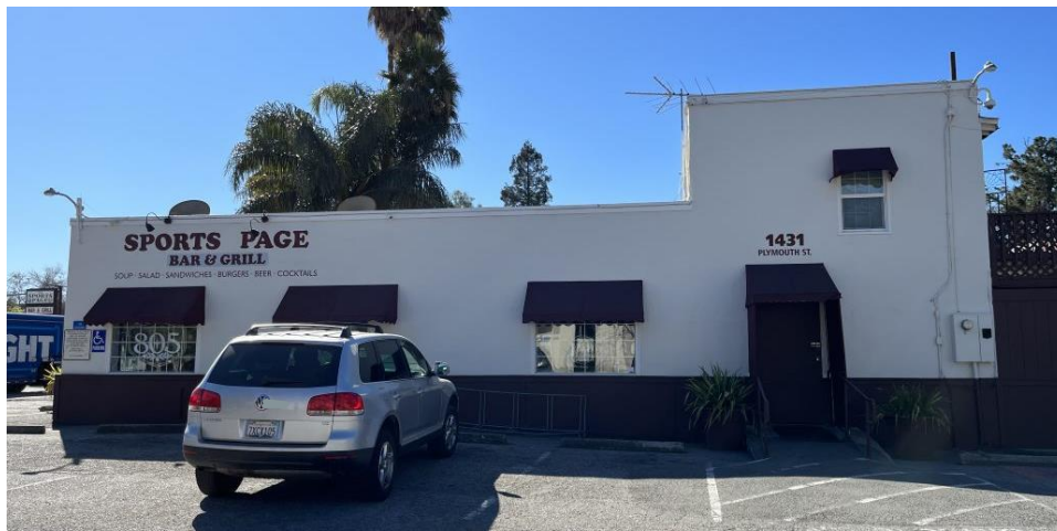
Figure 42. The north façade.
