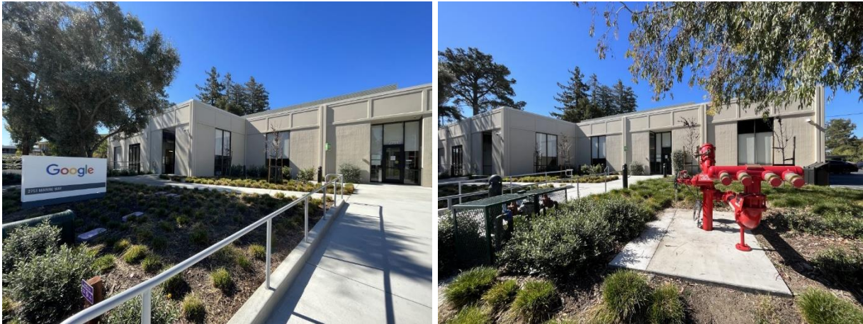
Figure 40. The east façade.
