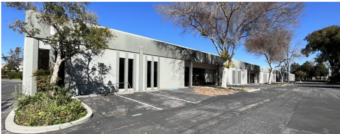
Figure 50. Building B, north façade.
