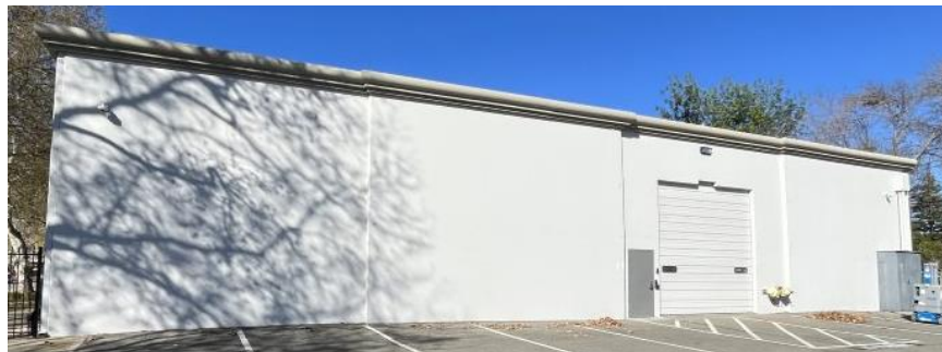
Figure 74. The west façade.
