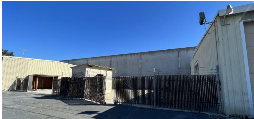
Figure 84. Two accessory structures between the buildings.
