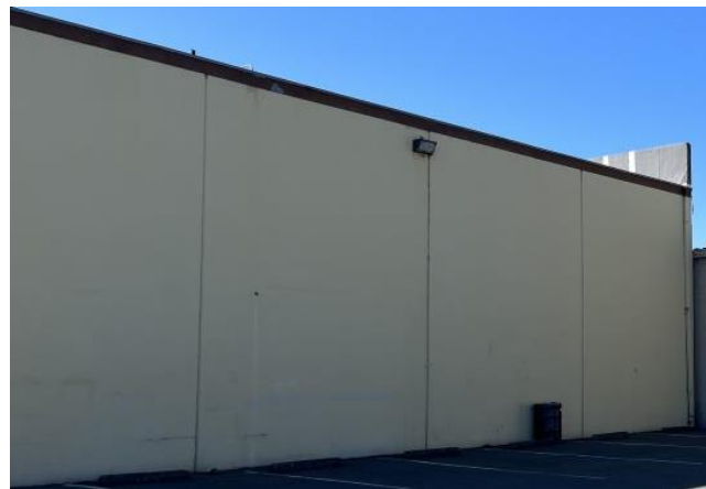
Figure 56. The north façade.
