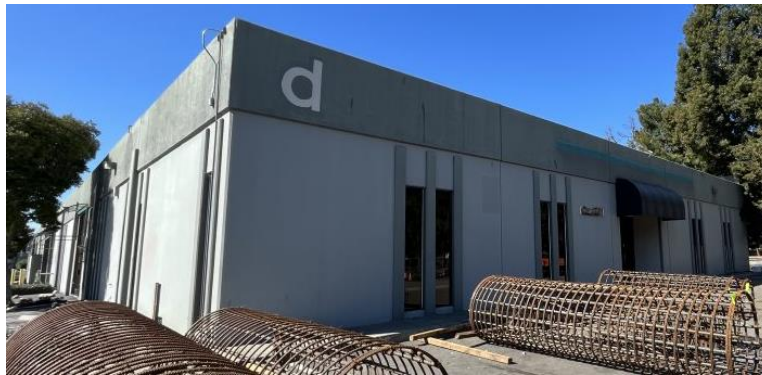
Figure 52. Building D, south façade.
