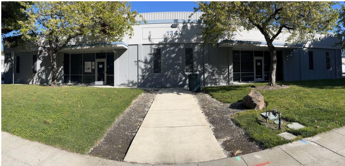
Figure 65. 1340 Space Park Way south façade.
