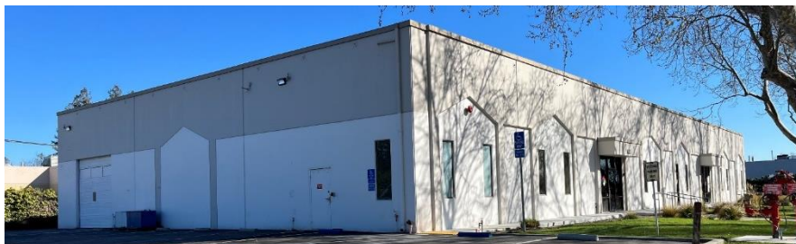
Figure 78. The east and south façades.
