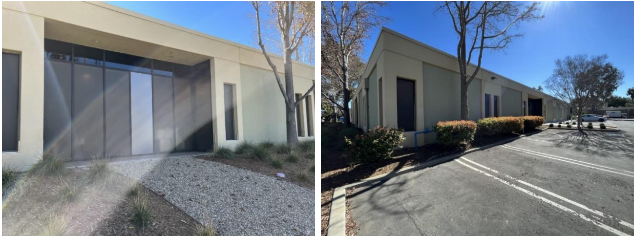
Figures 23 and 24. The north façade (left) and southeast corner of exterior (right).
