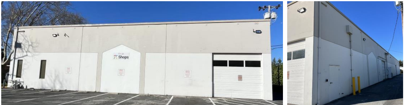
Figures 76 and 77. The west façade (left) and the north façade (right).
