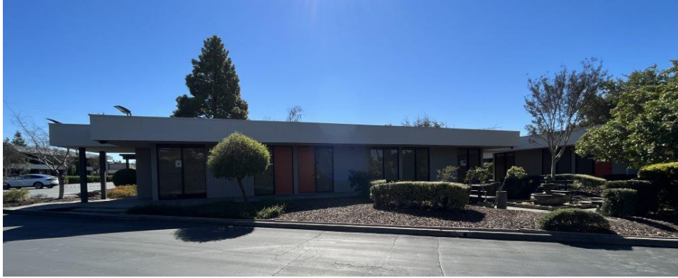
Figure 30. The east façade of the southeast building.
