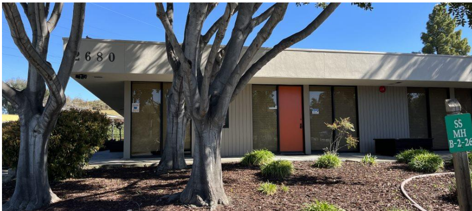
Figure 33. The north façade.
