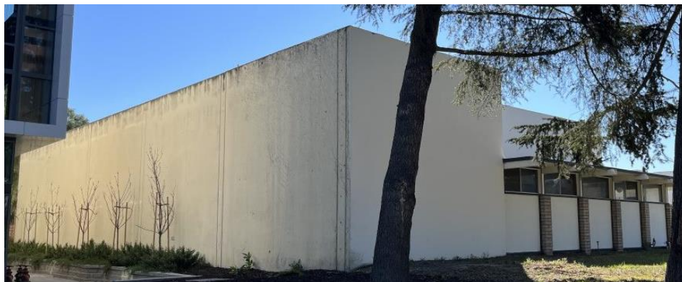
Figure 63. The north and west facades of 1601 N. Shoreline Boulevard.
