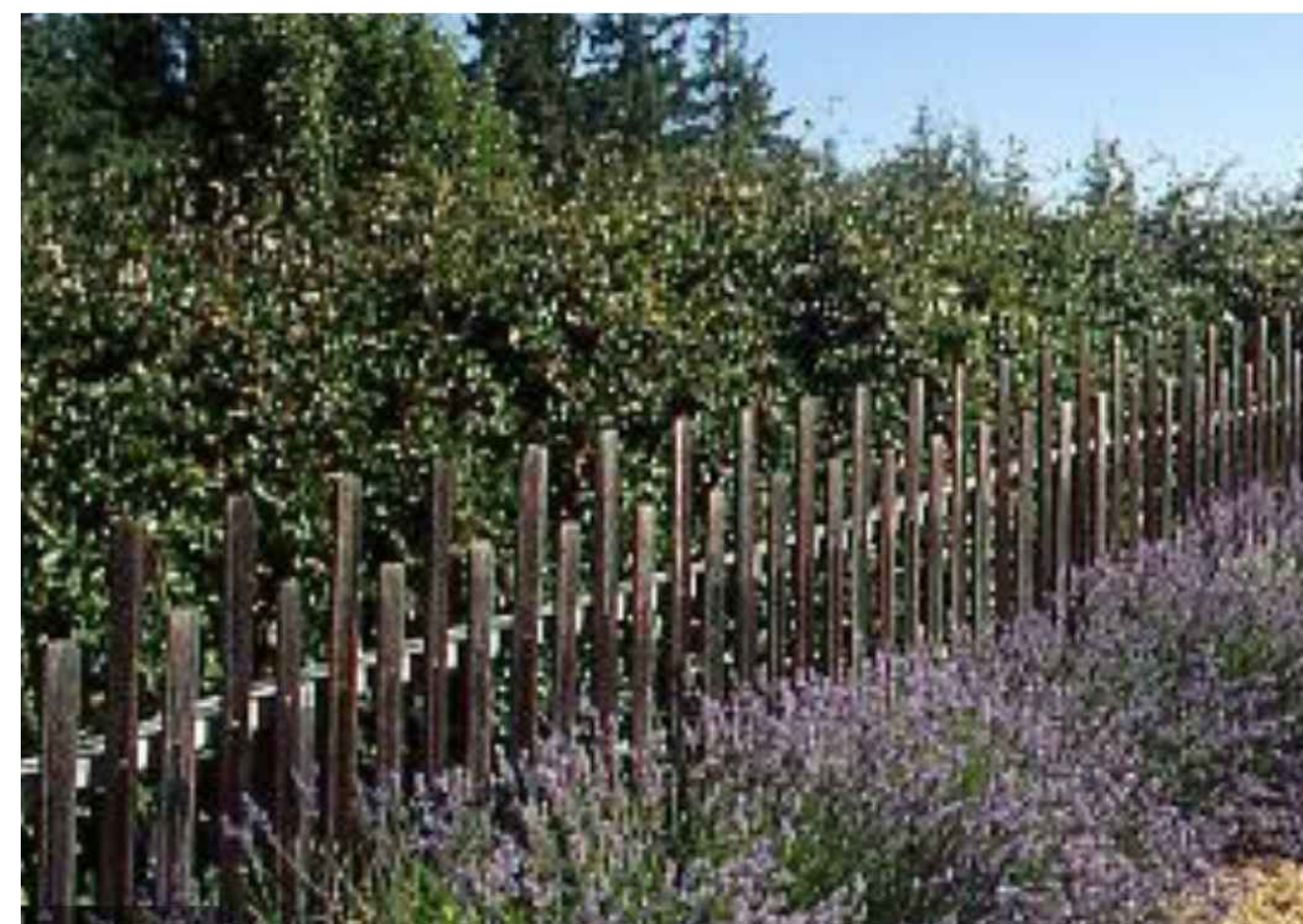
4 FEET TALL 2-3" ROUGH CEDAR OR REDWOOD GRAPE STAKES FENCE WITH 4" GAP BETWEEN GRAPE STAKES.
