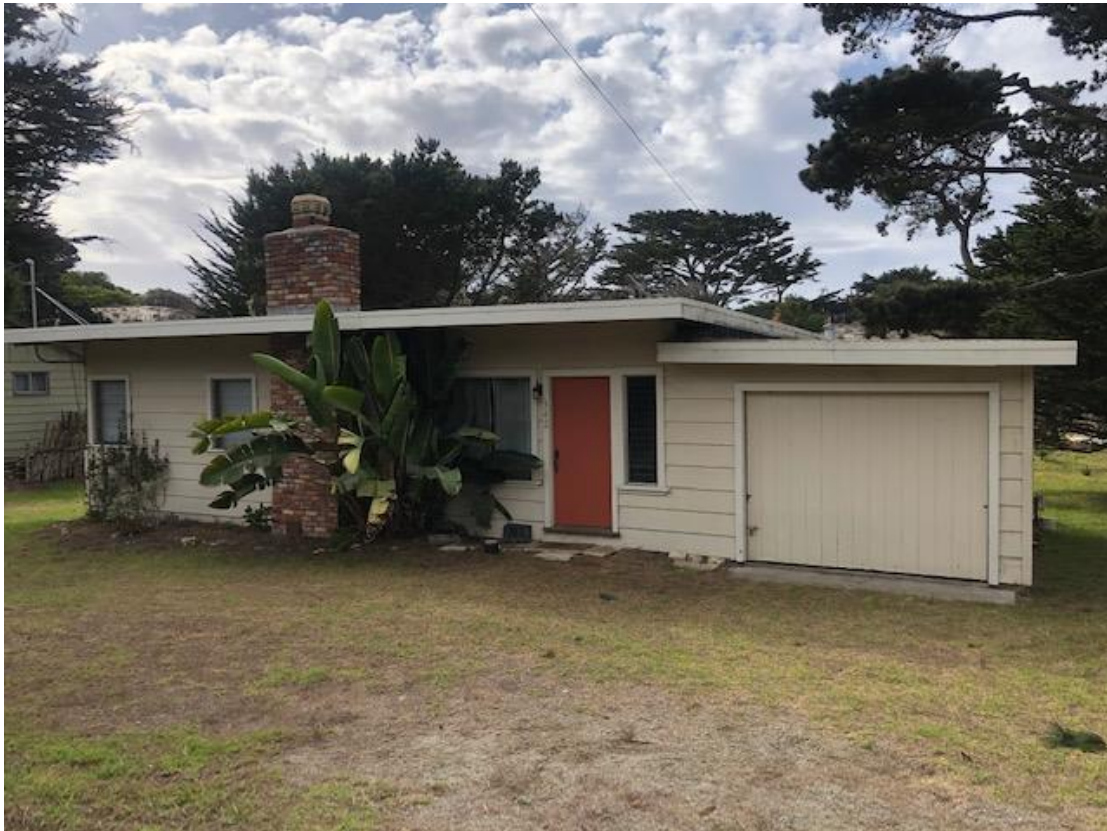
Figure 3: View of 342 Asilomar Boulevard, looking southwest.
