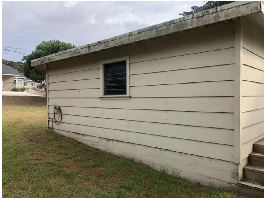
Photograph 6: View looking southeast at the north elevation of the residence.
