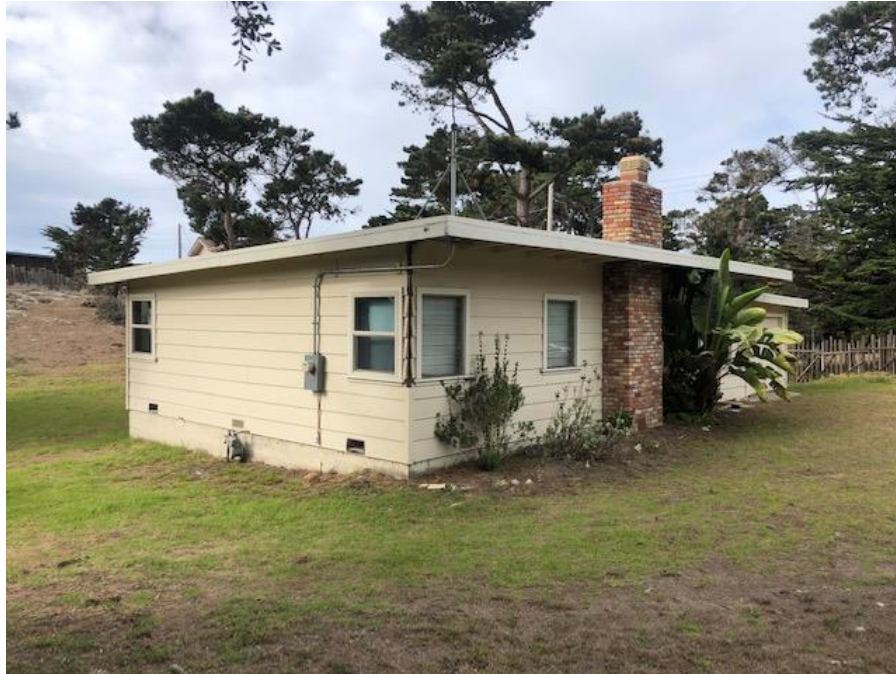
Photograph 3: View looking northwest at the southeast elevation of the residence with two replacement vinyl windows.
