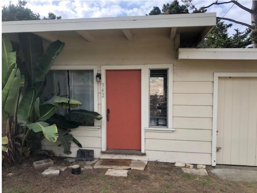
Photograph 1: View looking west at the front entry door, flanked by a louvered window on the right and fixed window on the left.
