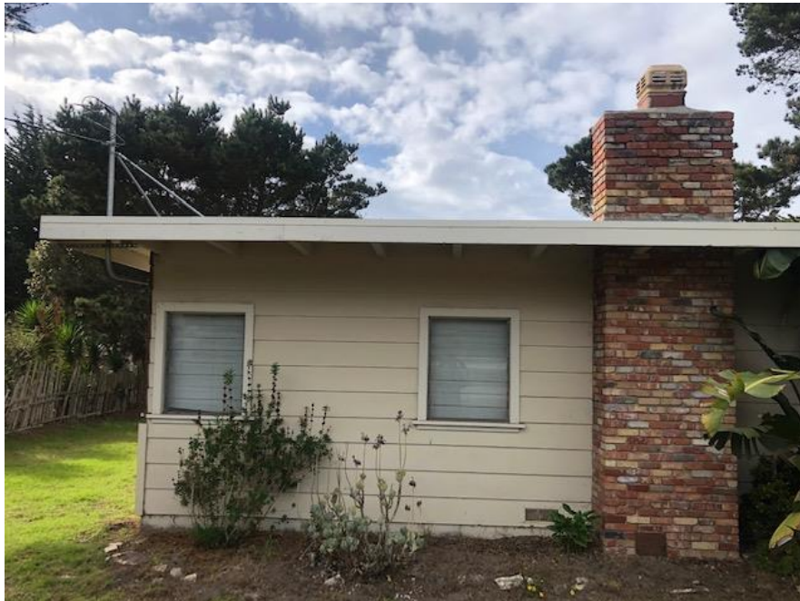
Photograph 2: View looking west at the left front of the residence with two louvered windows.
