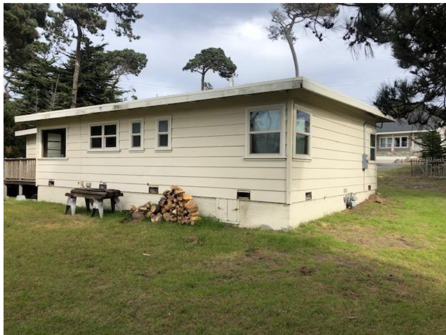
Photograph 4: View looking east at the southwest elevation of the residence. Note the replacement vinyl windows in the rear of the house.
