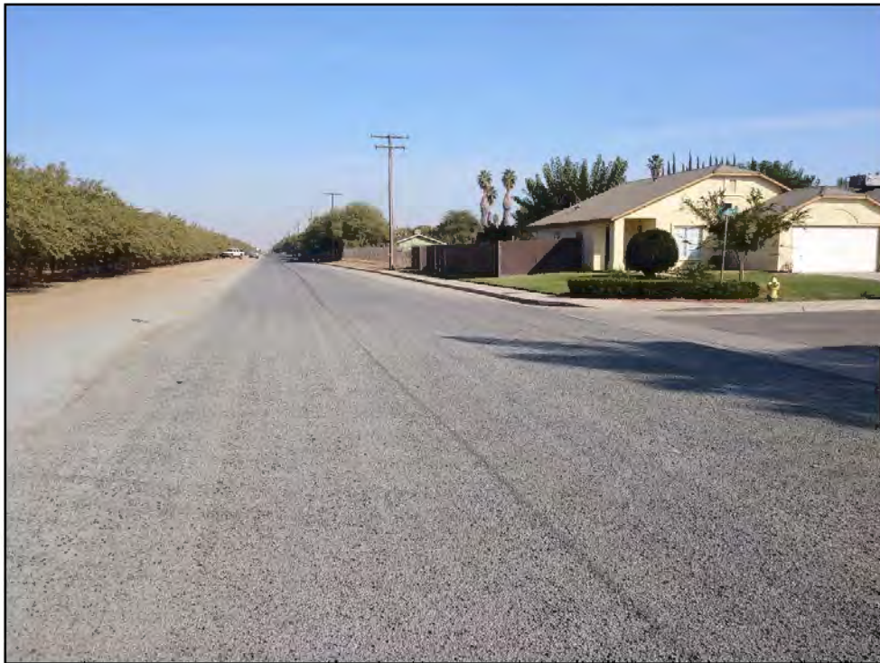
Figure 3. Overview of the proposed pipeline corridor along Road 164, looking north.
