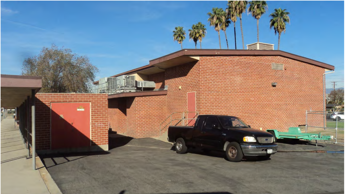
Photograph 7 – Looking west toward Multipurpose room from interior parking lot driveway.
