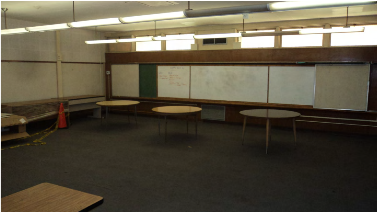
Photograph 12 – Classroom interior in Unit B.
