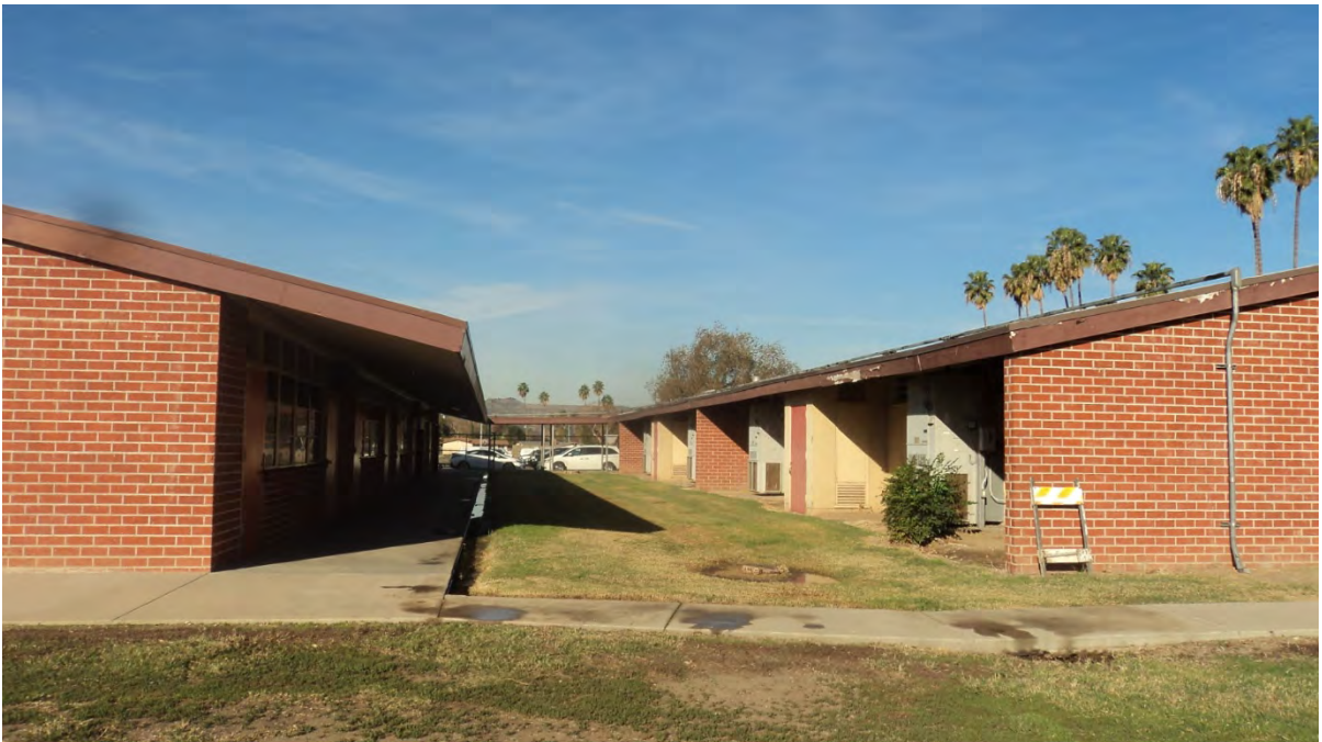
Photograph 10 – Looking east toward classroom buildings.
