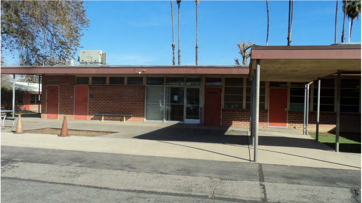
Photograph 9 – Looking north toward the central portion of the subject property and rear entrance to administrative offices.
