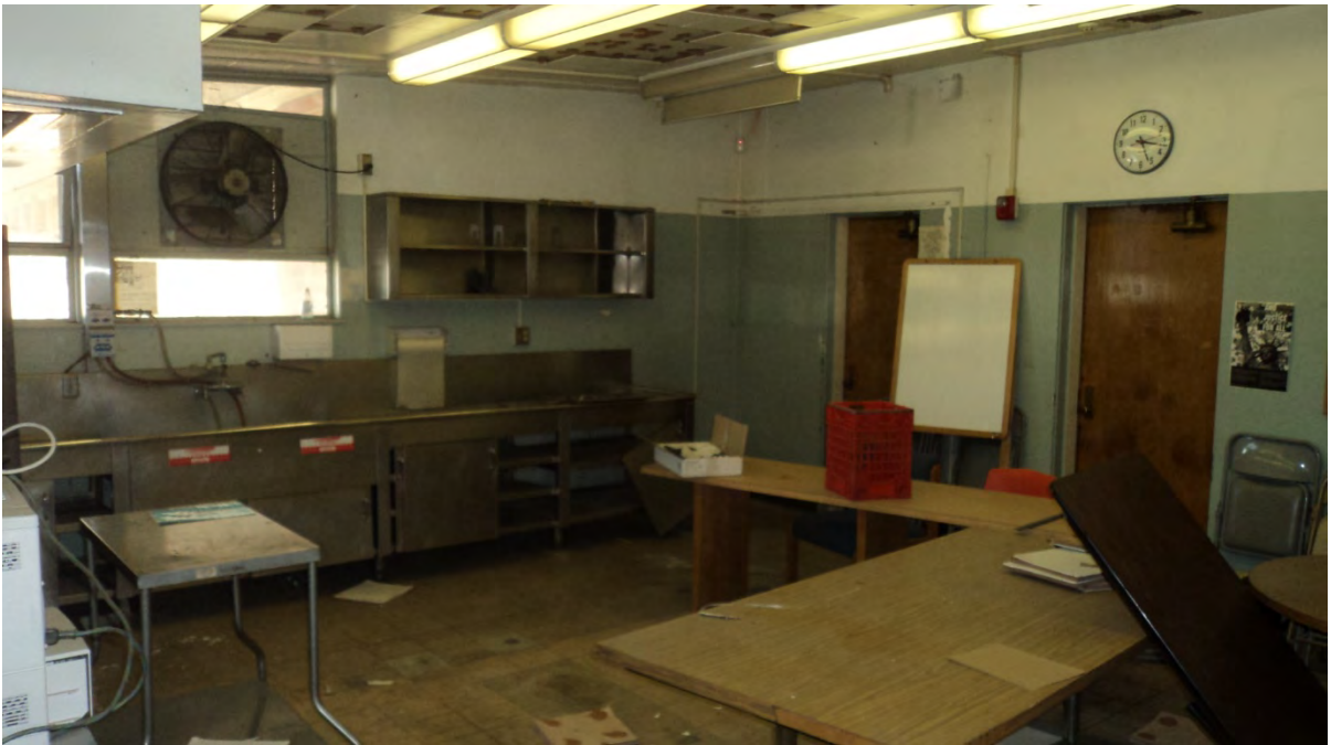
Photograph 16 – Cafeteria kitchen area adjacent to Multipurpose room.
