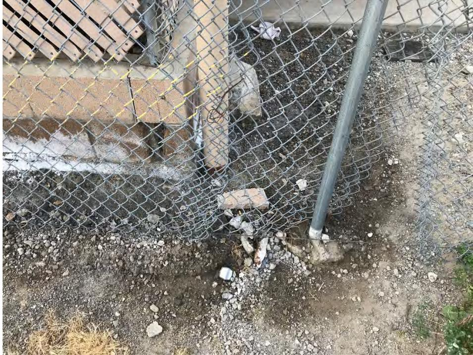
Photo 9 – The concrete containment wall was observed to be in poor condition, with some stained soil along the Property line. However, the staining is considered *de minimis* in nature.
