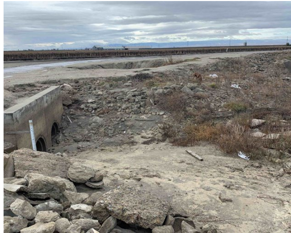
Photograph 4, Culvert at southeast corner of project site, facing southwest.
