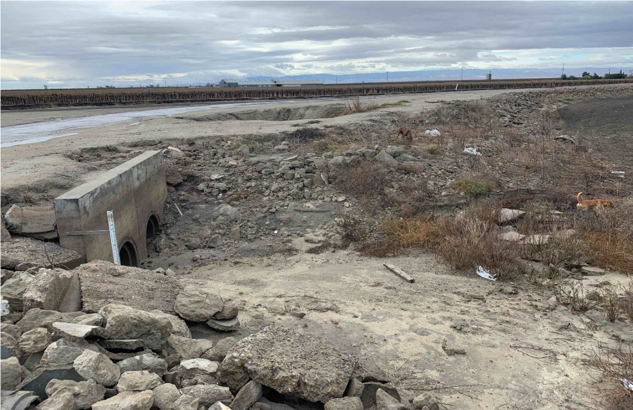
Photograph 4. Culvert at southeast corner of project site, facing southwest.
