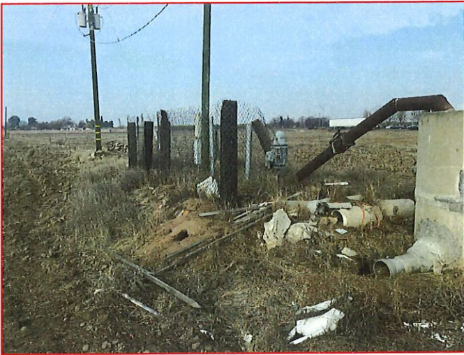
IRRIGATION PIPING, AND POWER POLES LOCATED IN THE CENTER OF THE SITE.
