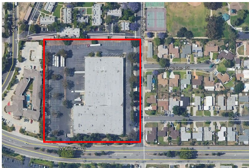
Figure A-8 Warehouse Site
