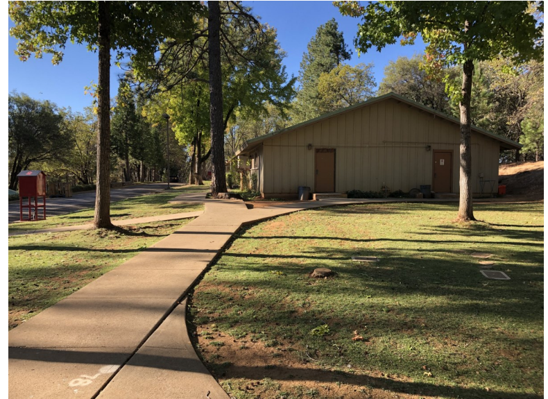
View of existing inmate barracks from mess hall/kitchen.
