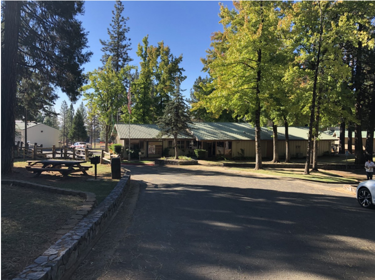
View of existing administration building, looking south from entrance driveway.
