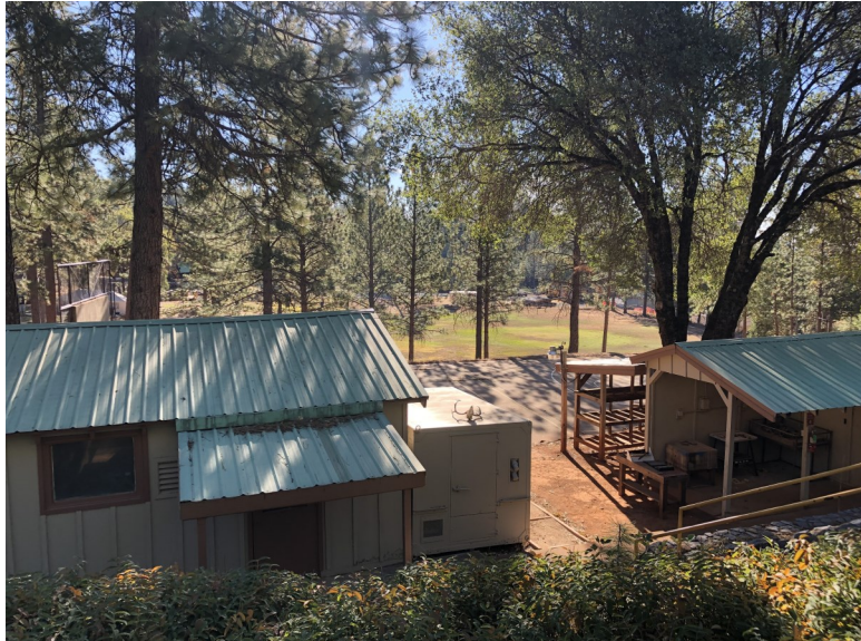
View of existing utility buildings east of inmate barracks.
