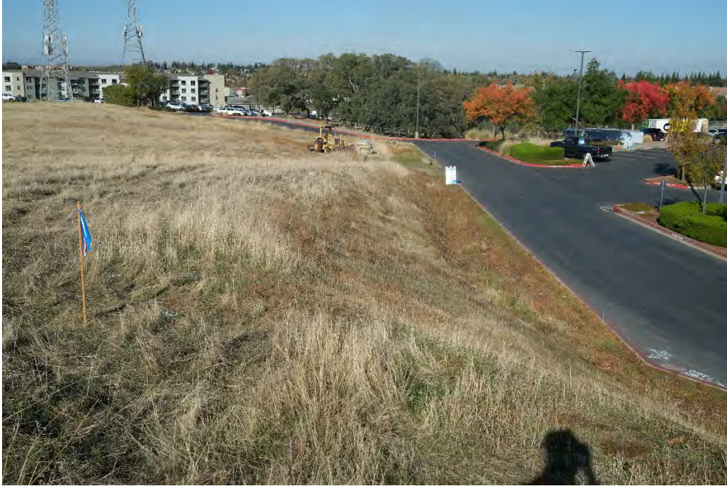
Photo 3. Closeup of steep slope below Lot 1's northeast corner, facing northwest.
