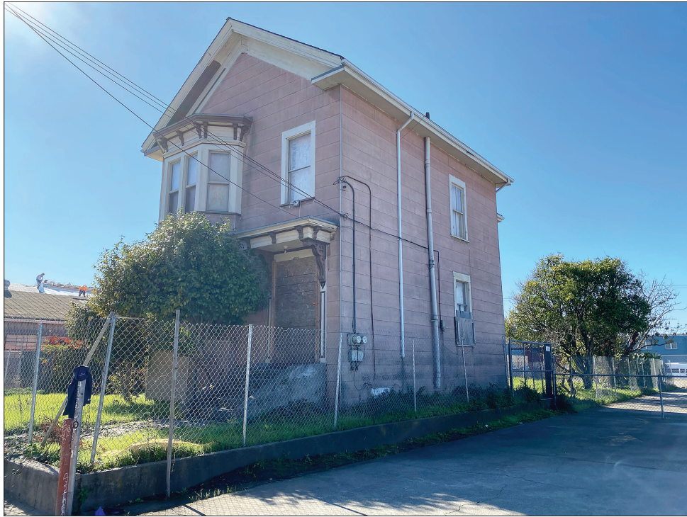
Photo 1: Existing residential duplex building at 2212 Fifth Street, as seen from Fifth Street
