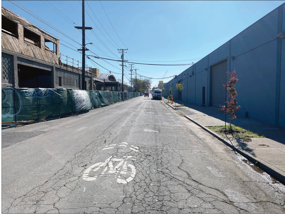
Photo 3: Existing warehouse building at 747 Bancroft Way, as seen from Fourth Street
