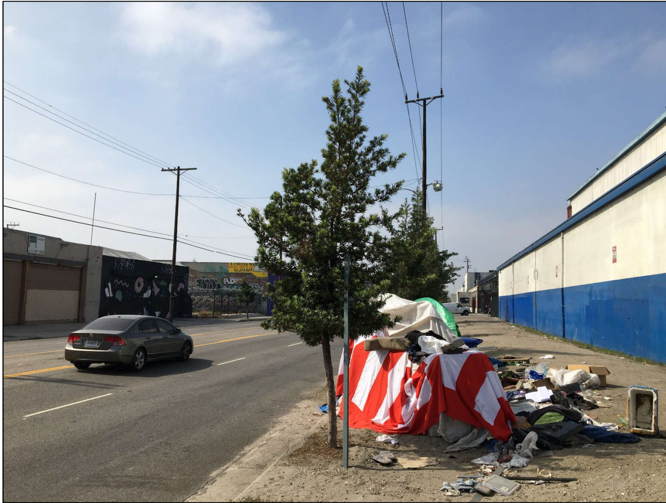
Photo 16 (South). Tree Number 16. Removal required to accommodate construction.
