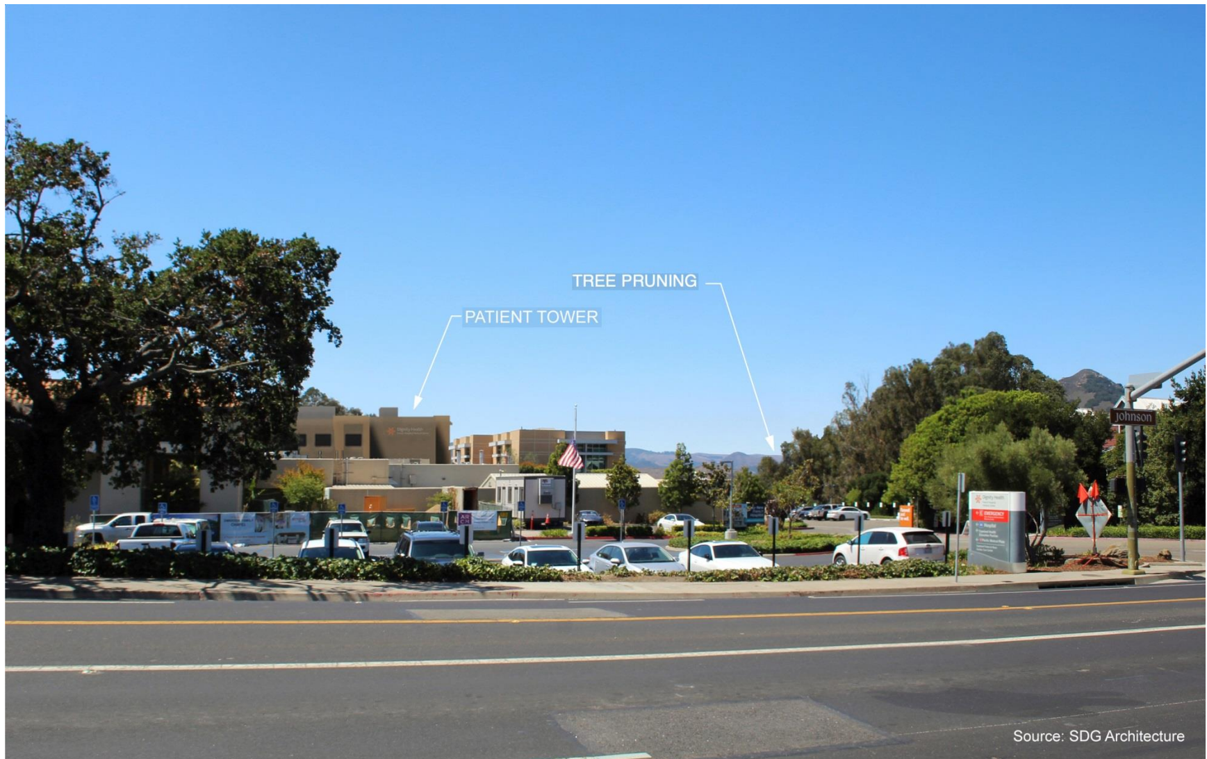
KVA-2 - From Johnson Avenue looking west
