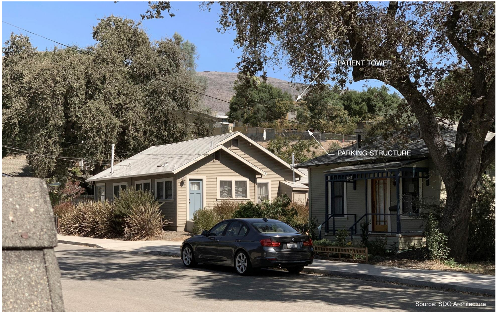
KVA-8 - From Leff Street looking east.
