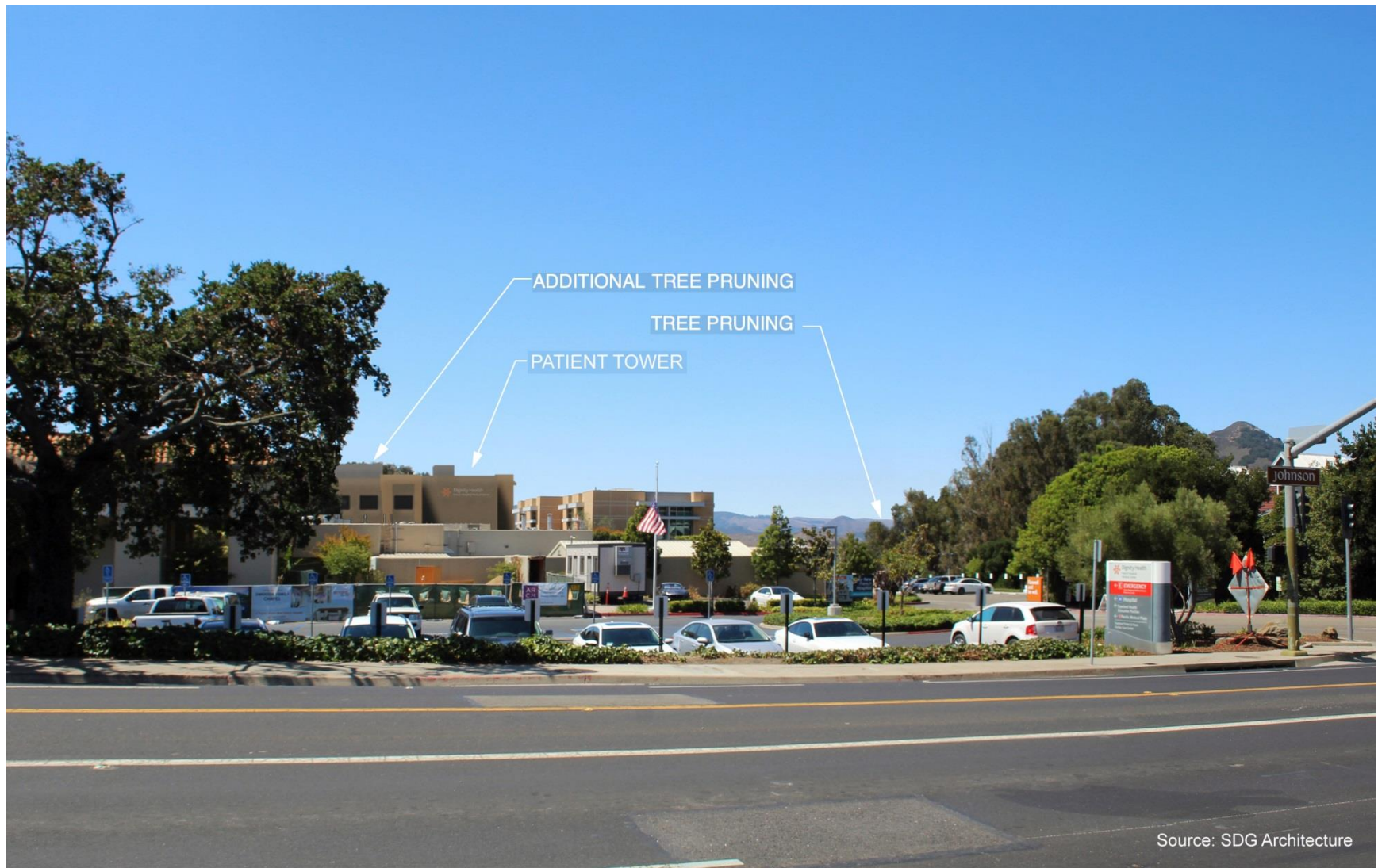
KVA-2 - From Johnson Avenue looking west
