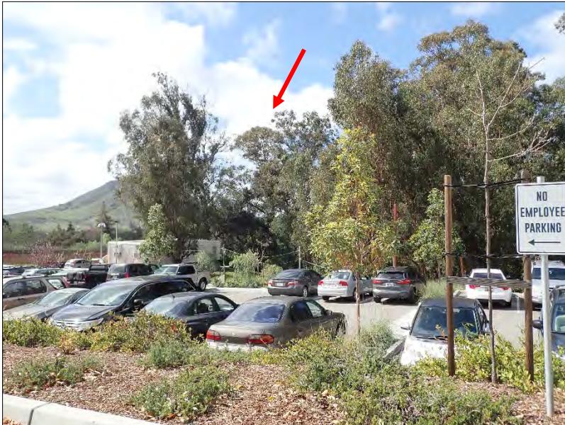
Photo 1: View southwest at eucalyptus removal "north" area (arrow) around construction trailer at the edge of the parking lot. 4/17/2021
