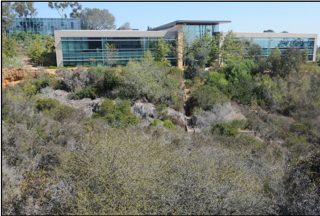
PHOTOGRAPH 1 View of Survey Area, Looking North Note Stairway
