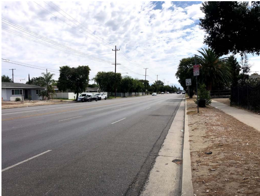
Plate 1: Overview of paved APE along Roscoe Boulevard near Mason Avenue (View: East)
