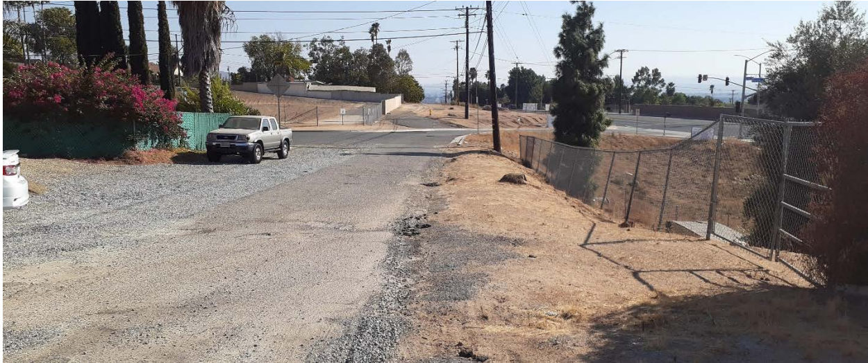
Photograph No. 1: Current street conditions at Judson St. towards Perris Blvd, facing south
