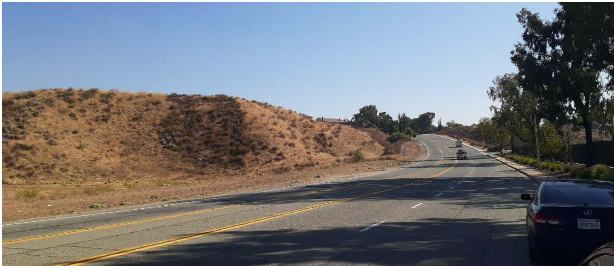
Photograph No. 4: Current street conditions on Perris Blvd. towards Canyon Vista Rd., facing south.
