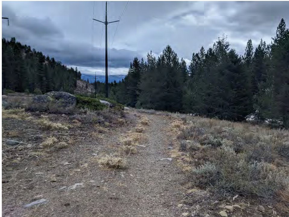
Photo 2: View of the proposed pipeline location passing beneath existing overhead electrical transmission lines in the eastern portion of the Study Area. Photo taken October 13, 2021.
