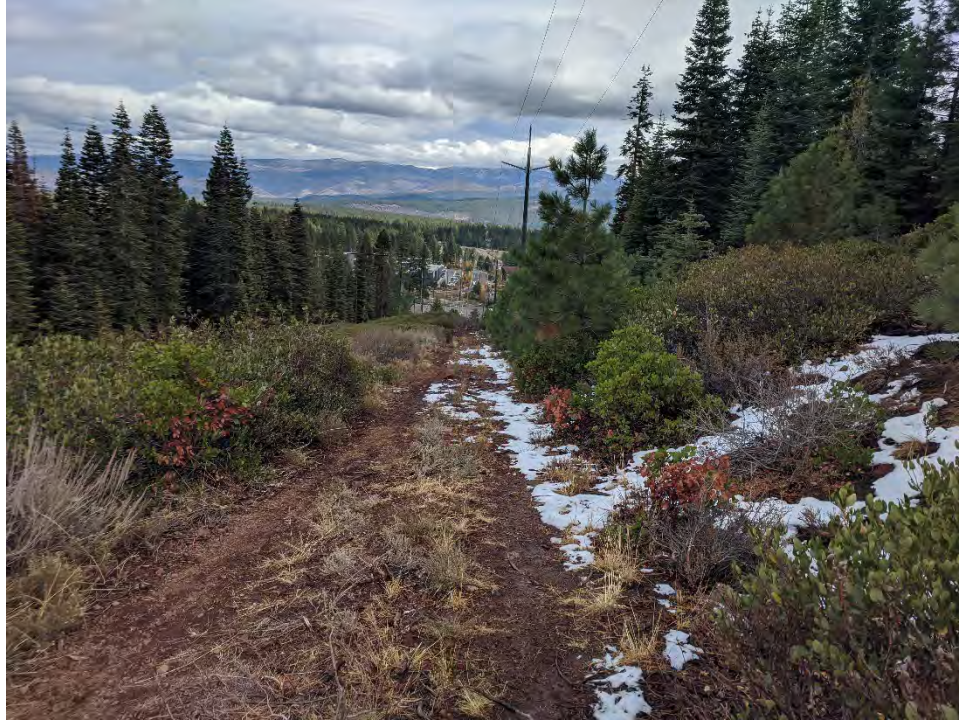
Photo 7: View of the proposed pipeline location passing beneath existing overhead electrical transmission lines. Photo taken October 13, 2021.
