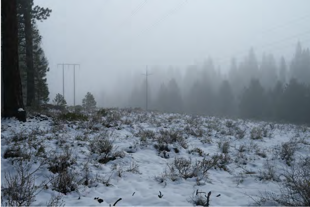
Photograph 3. Proposed Alignment B along the existing overhead utility corridor, looking east.
