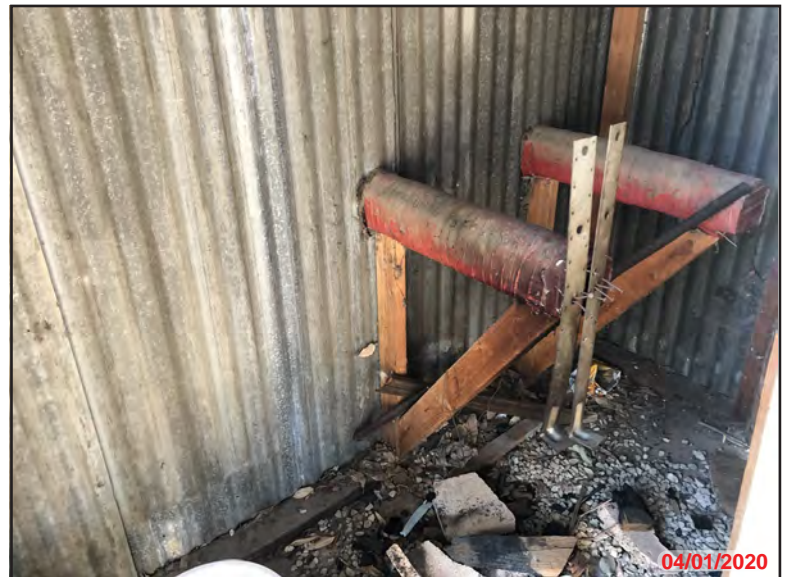
Photo 24 - Exterior APN: 289-220-004, northerly exterior face of maintenance shed.
