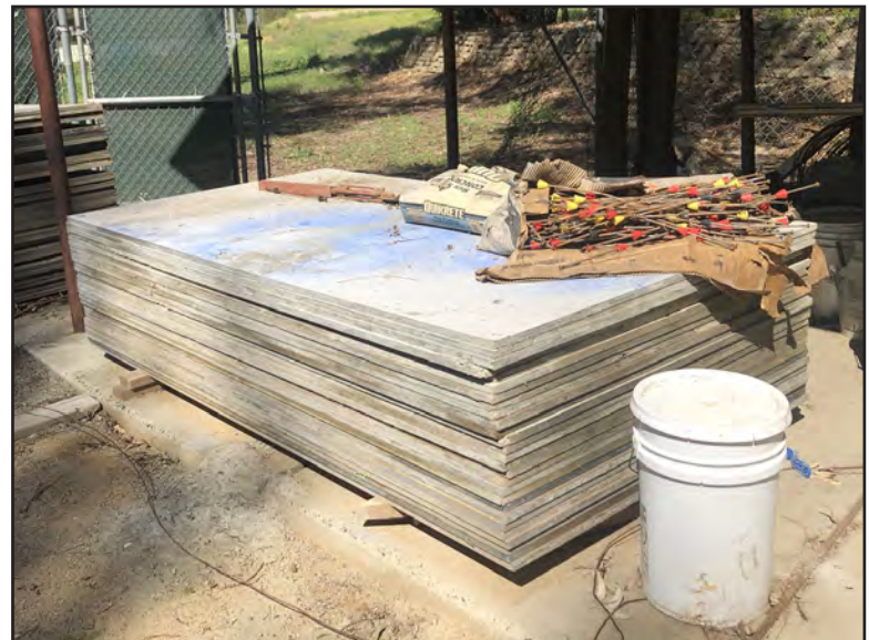
Photo 20 - Exterior APN: 289-220-004, Northeast corner of Target Property south of APN:289:220-003 and south of apparent storage/ maintenance shed at stack of plywood and misc. construction debris.
