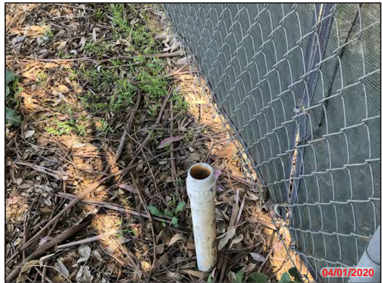
Photo 36 - Exterior APN: 289-220-005, apparent irrigation line located near southeasterly Target Property line. Does not appear to be a vent pipe for subterranean structure.
