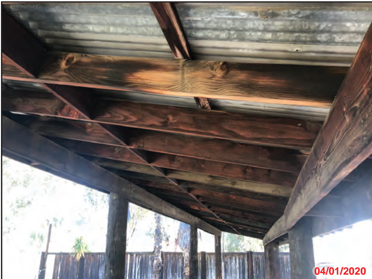
Photo 11 - Exterior APN: 289-220-003, under canopy with top interior ceiling in view.
