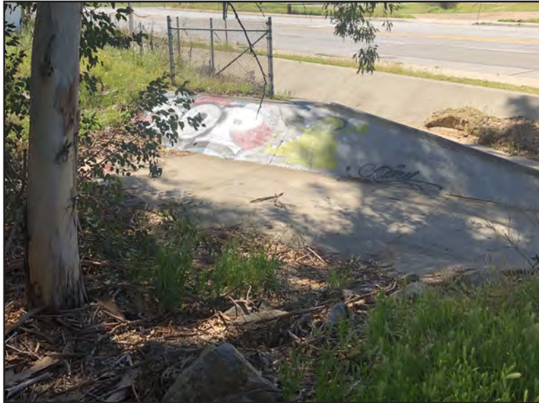
Photo 45- Exterior APN: 289-220-006, drainage basin at southeast Target Property boundary.
