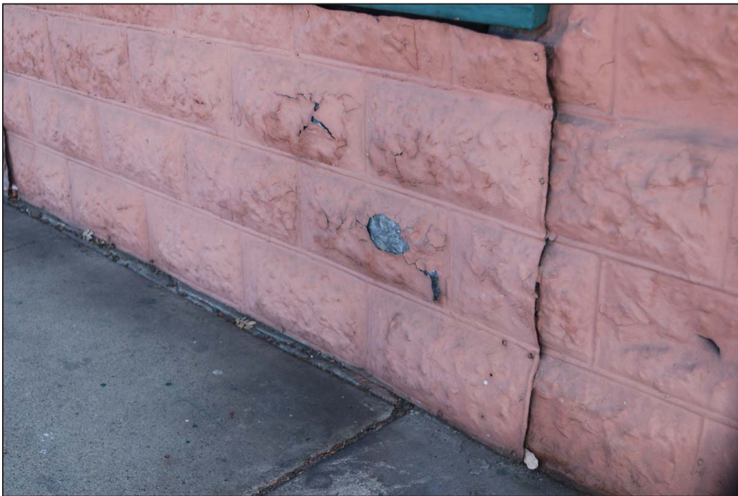
Photo 36: West elevation, condition of pressed tin
