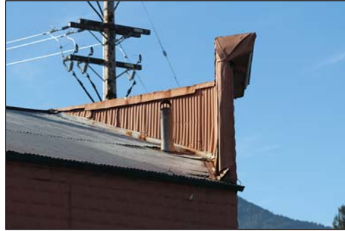
Northwest corner, False Front Detail
