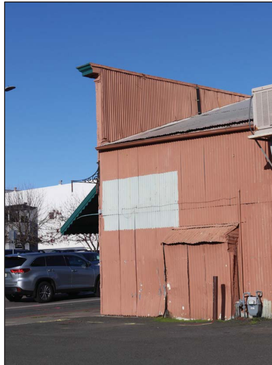
Photo 38: West elevation false front (looking NW)
