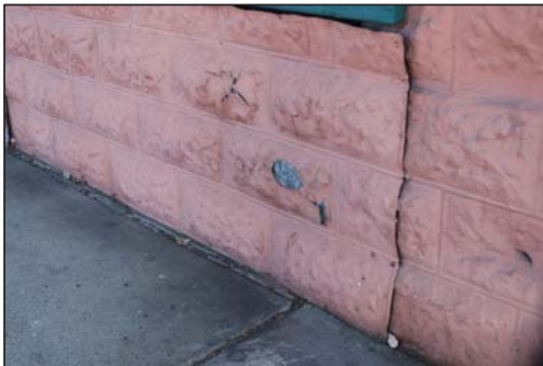
West Elevation, Pressed Tin Detail
