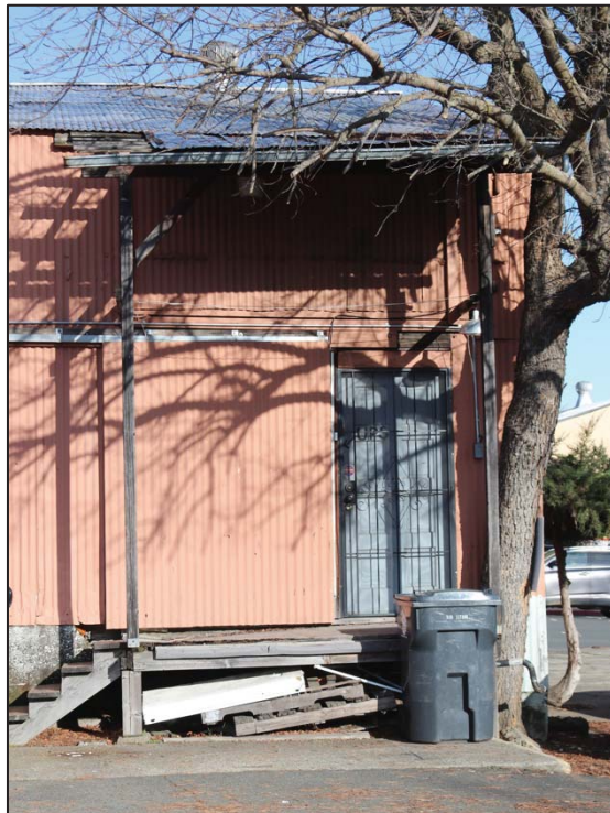
Photo 42: South elevation, pedestrian entrance at SE corner
