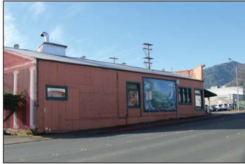
North Elevation (Perkins Street)
