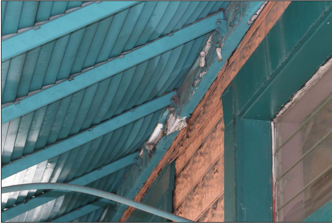
Photo 35: West elevation, ceiling of awning
