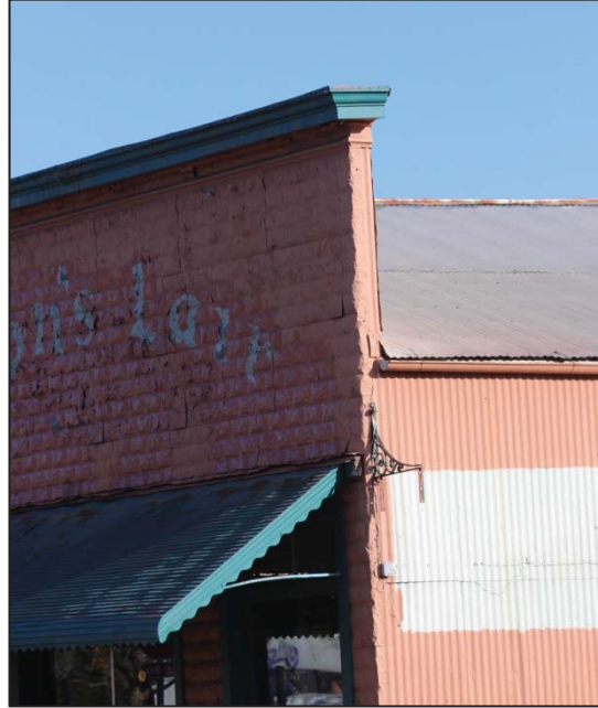
Photo 37: West elevation, false fronting (looking NE)
