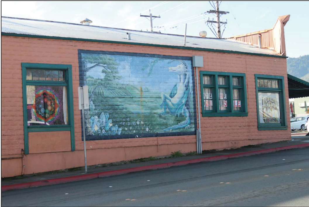
Photo 47: North elevation, mural and windows
