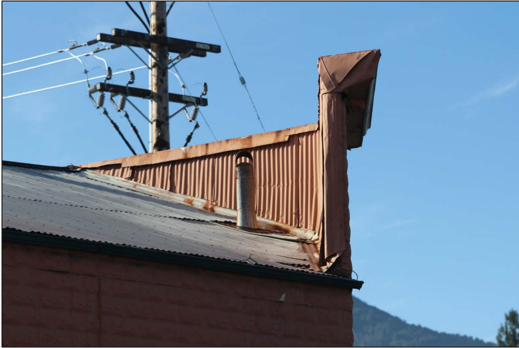
Photo 39: West elevation, false front (looking SW)
