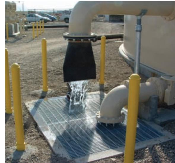
Municipalities are challenged with protecting water storage tanks against contamination. Insects, rodents, birds, or tampering can cause serious health risks. Tideflex® Check Valves provide a reliable, cost-effective and maintenance-free solution compared to screens and flap valves.
