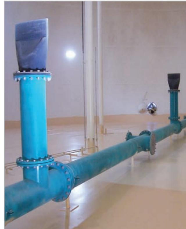
In circular, rectangular and irregularly-shaped reservoirs, the diameter or length is greater than the depth. A single fixed-diameter inlet pipe (common or separate from outlet pipe) results in short-circuiting, poor mixing and dead zones in areas away from the inlet because the momentum is concentrated in one localized area of the tank.
