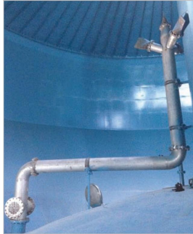
Elevated tanks are prone to poor mixing in summer and icing in winter, due to a large surface area exposed to the sun and the elements. The inlet-outlet pipe of Sphere-Spheroid, Fluted-Column and Composite Elevated Tanks (CET) runs up the pedestal, or dry riser, and penetrates the bottom of the bowl.
