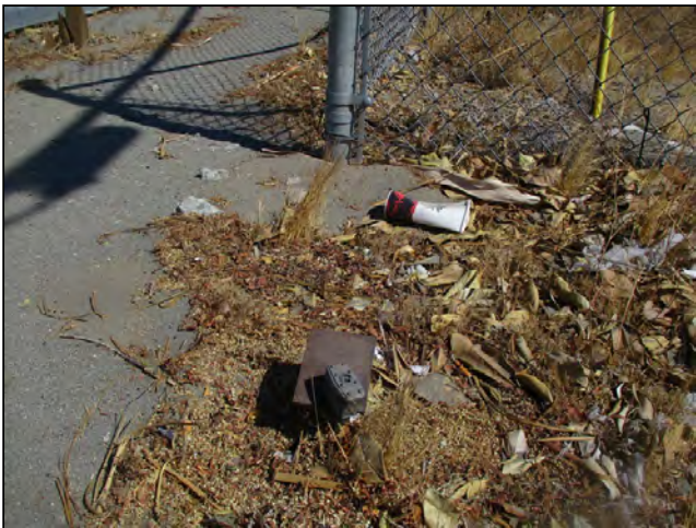
Apparent locked below ground structure near Temescal Wash, south.
