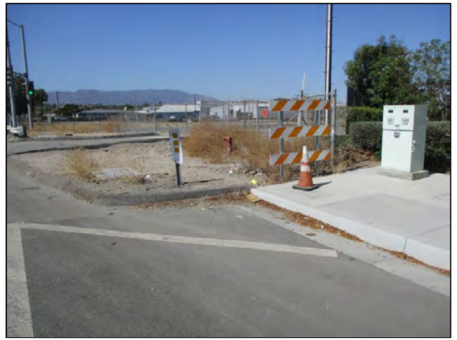
Area of bridge widening along north side near Temescal Wash
