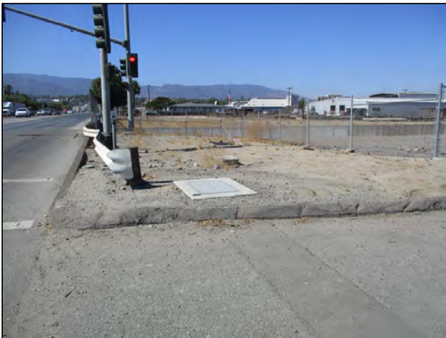
North area of impact at Temescal Wash
