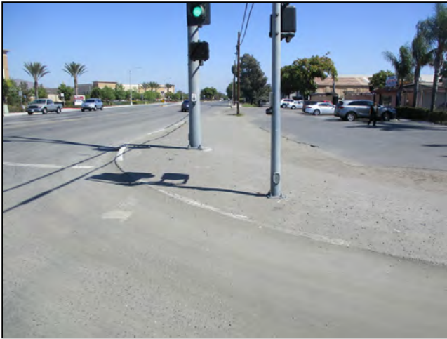
View of sidewalk and portion of parking lot in front of Corona Auto Parts
