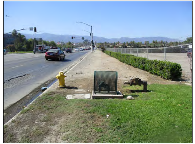
Dirt sidewalk on north side of Project Area adjacent to Clow Valve
