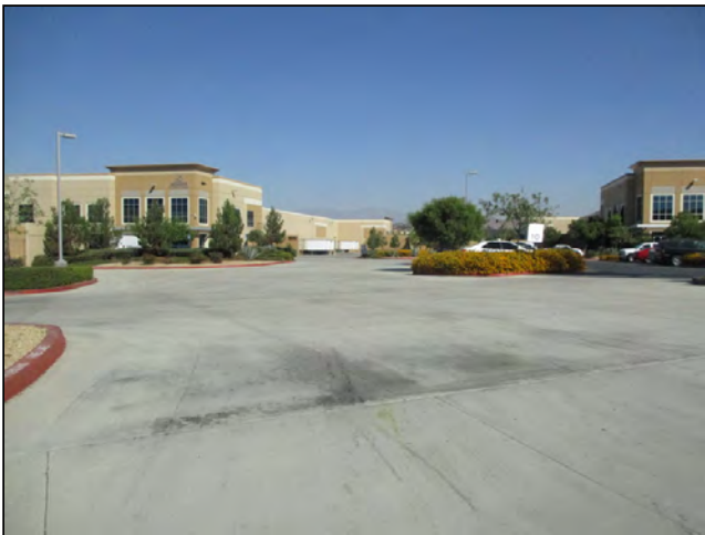
North adjacent properties
