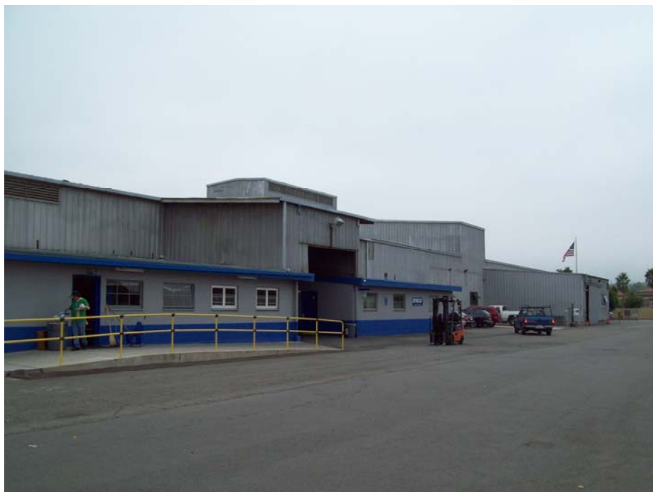
Photograph 3: Northwest-facing entrance of L-shaped building, camera facing southwest, September 13, 2011
