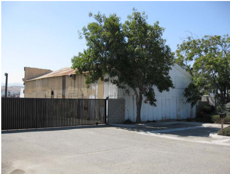
Photograph 2: Northwest building, northeast and northwest elevations, camera facing southwest, September 13, 2011
