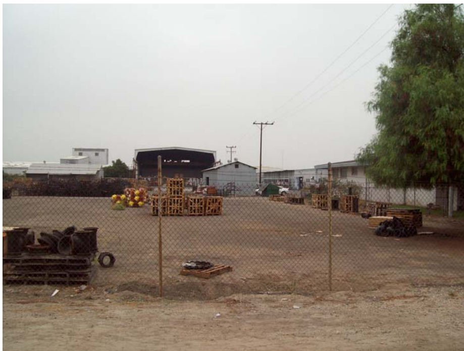
Photograph 5: Southern open-sided bay of L-shaped building at center rear, smaller utilitarian buildings at center and left, southwest elevation of office building at right, camera facing northwest, September 13, 2011
