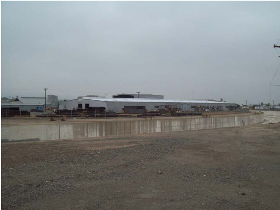
Photograph 2: South wing of L-shaped building, camera facing northwest, September 13, 2011
