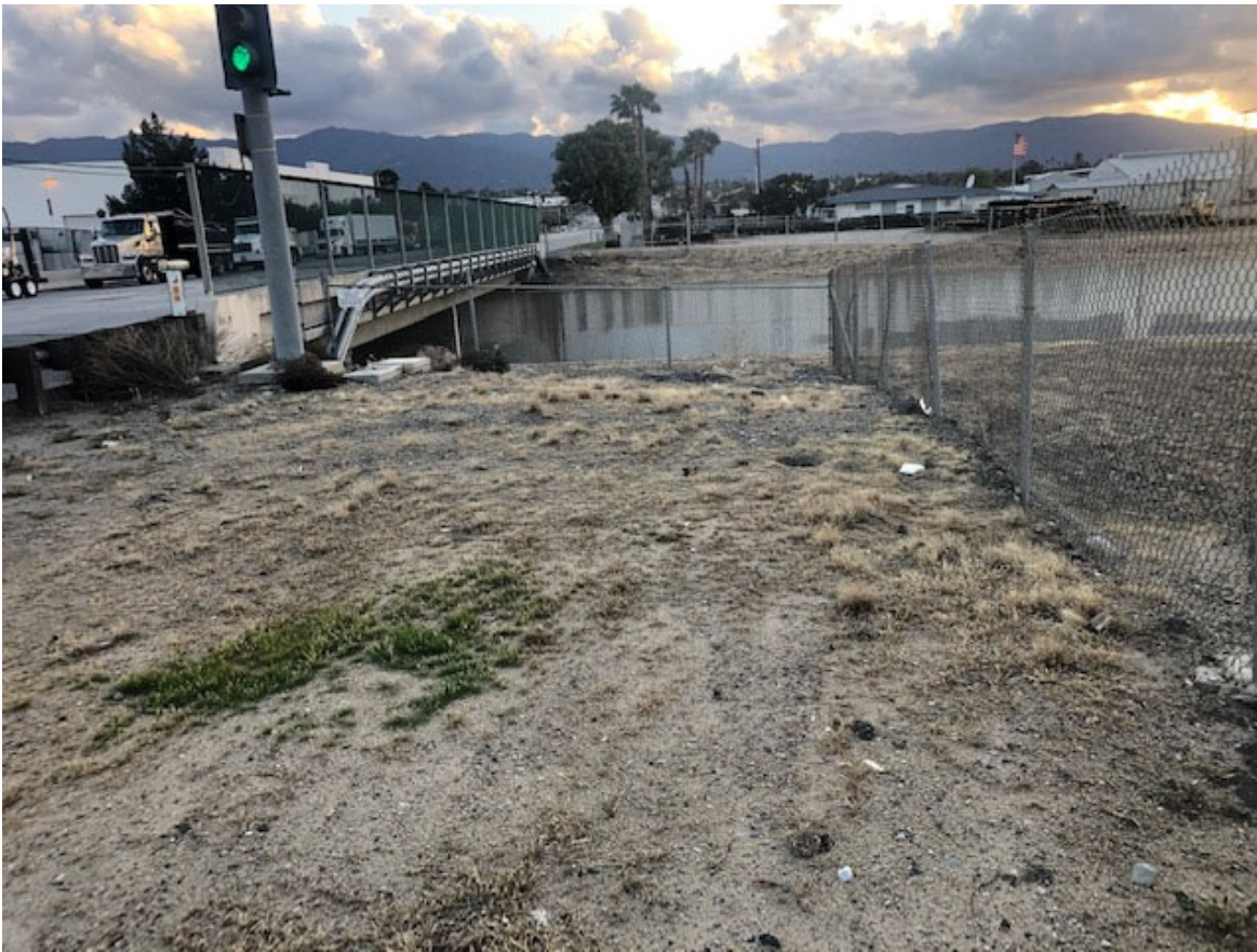
Photo 3. Looking west from the northern side of the concrete wash.
