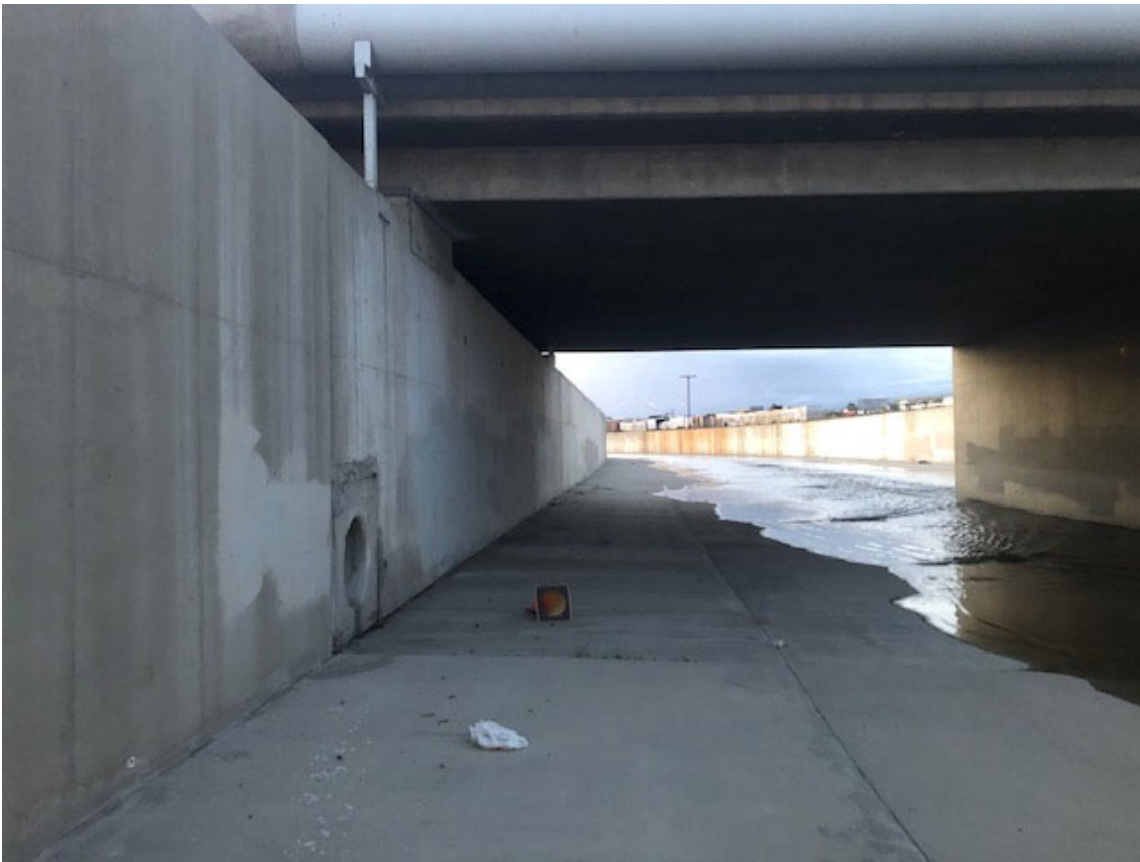
Photo 5. Looking north down in the concrete wash.
