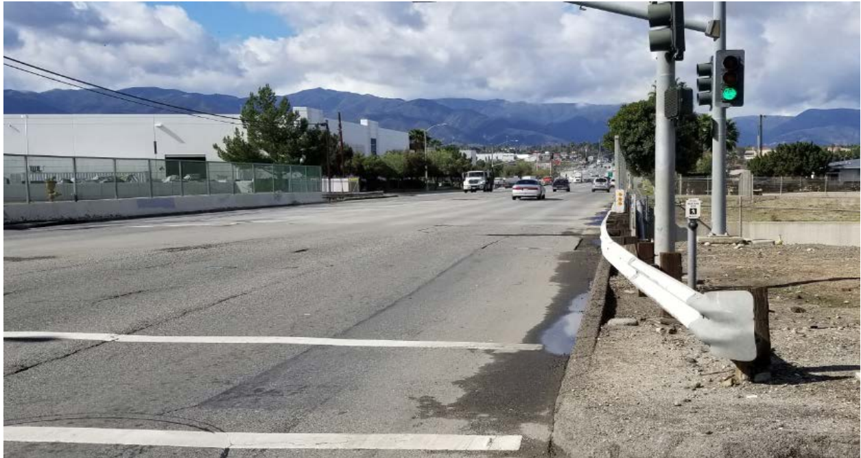
Photograph No. 2, Magnolia Avenue Bridge, facing southwest.
