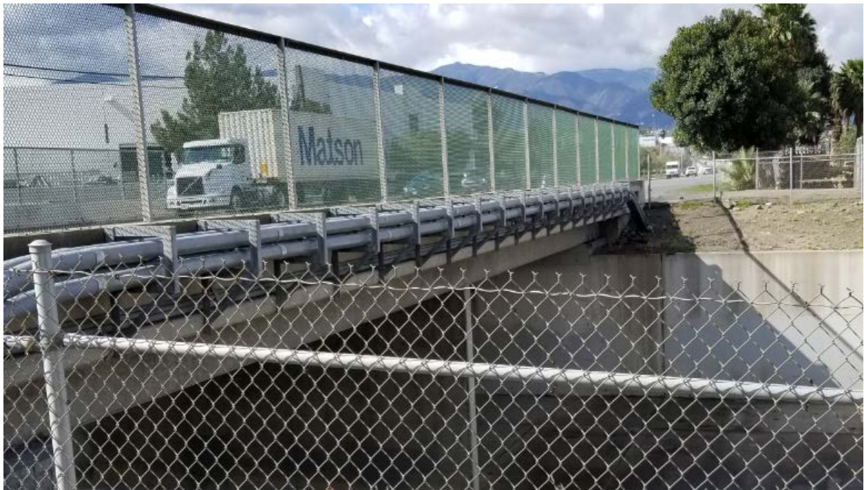
Photograph No. 3, Northwest side of the bridge.
