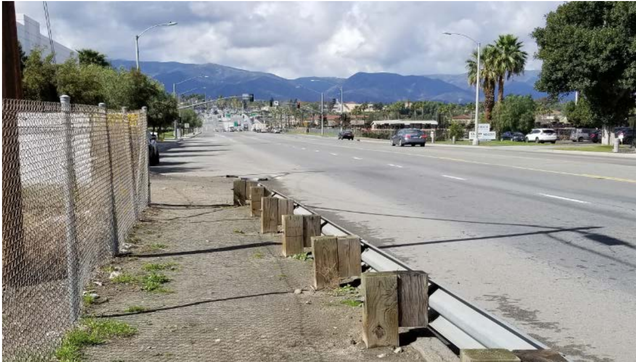
Photograph No. 4, Magnolia Avenue, southwest of the bridge.
