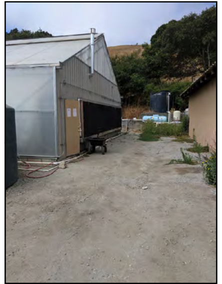
Looking west at access road between existing greenhouses and residence.
