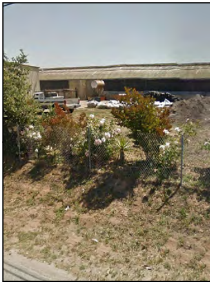
Looking northeast at existing greenhouses and parking from McGinnis Road.
