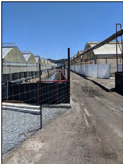
Looking west at access road and existing greenhouses.
